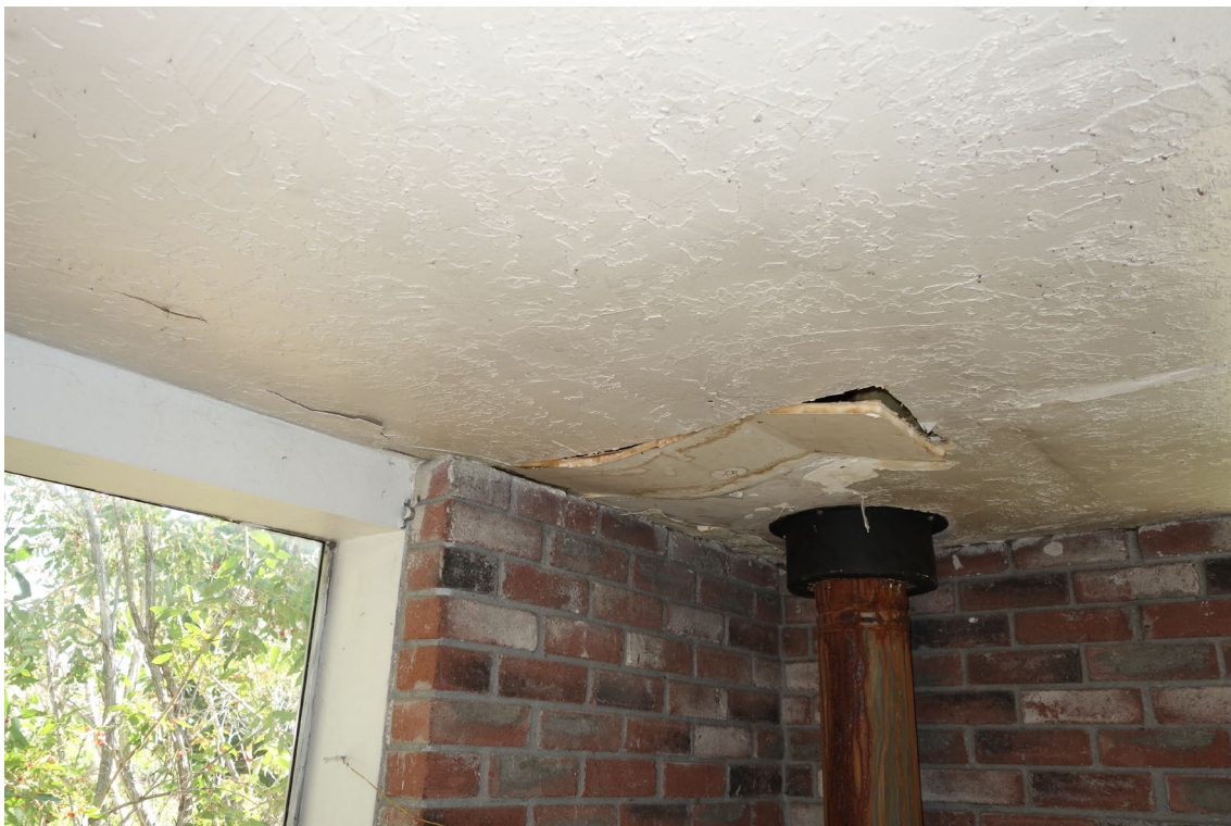
Nursery Cook House - Building #0890 Description: Roof Replacement & Drywall Repairs Needed.
