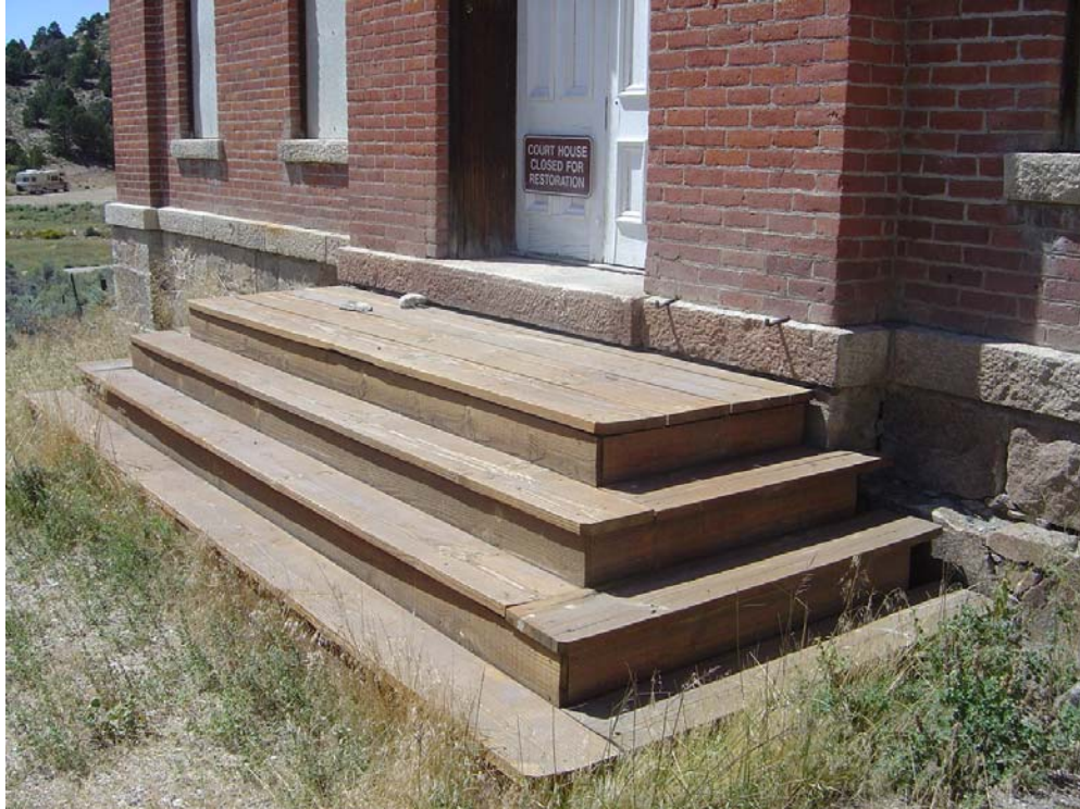
Belmont Courthouse - Building #0999 Description: Front steps to the courthouse.
