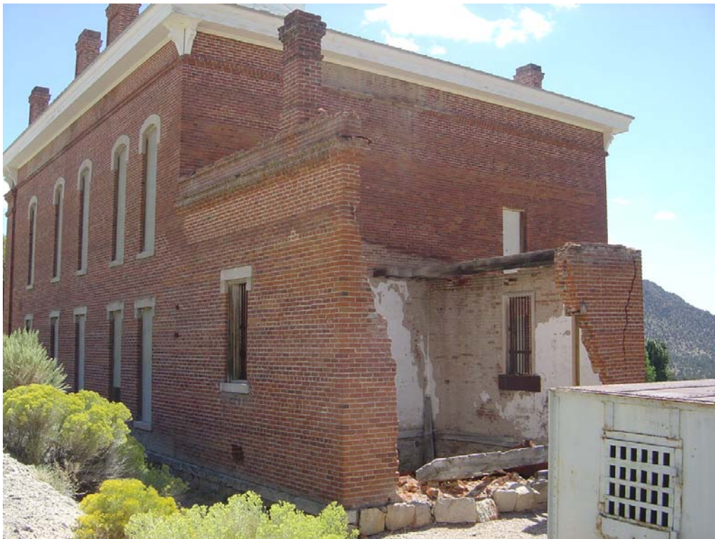
Belmont Courthouse #0999 Description: Rear view of the courthouse.
