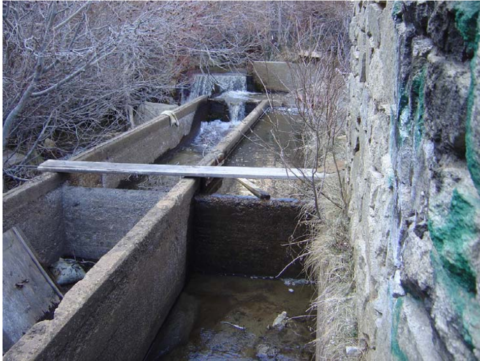
Stewart Irrigation Diversion Building - Building #2451 Description: Concrete diversion channels.
