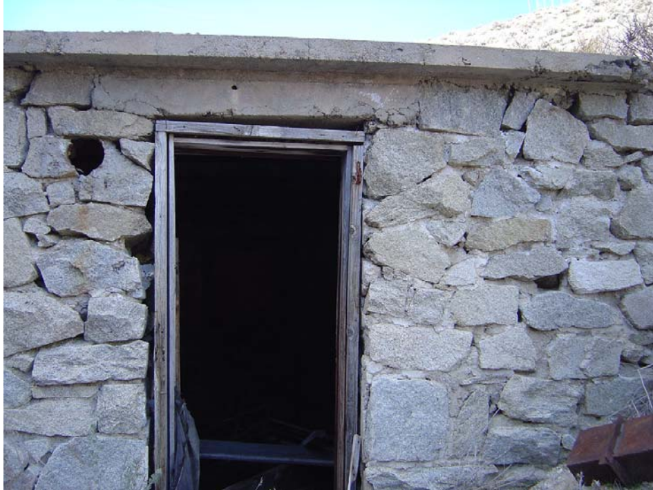
Stewart Irrigation Diversion Building - Building #2451
