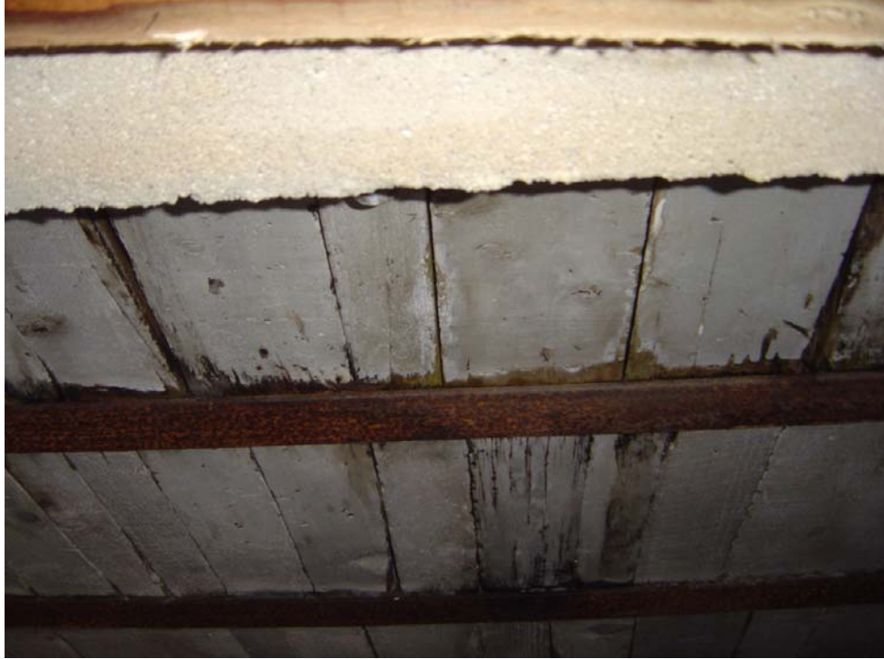
Stewart Irrigation Diversion Building - Building #2451
