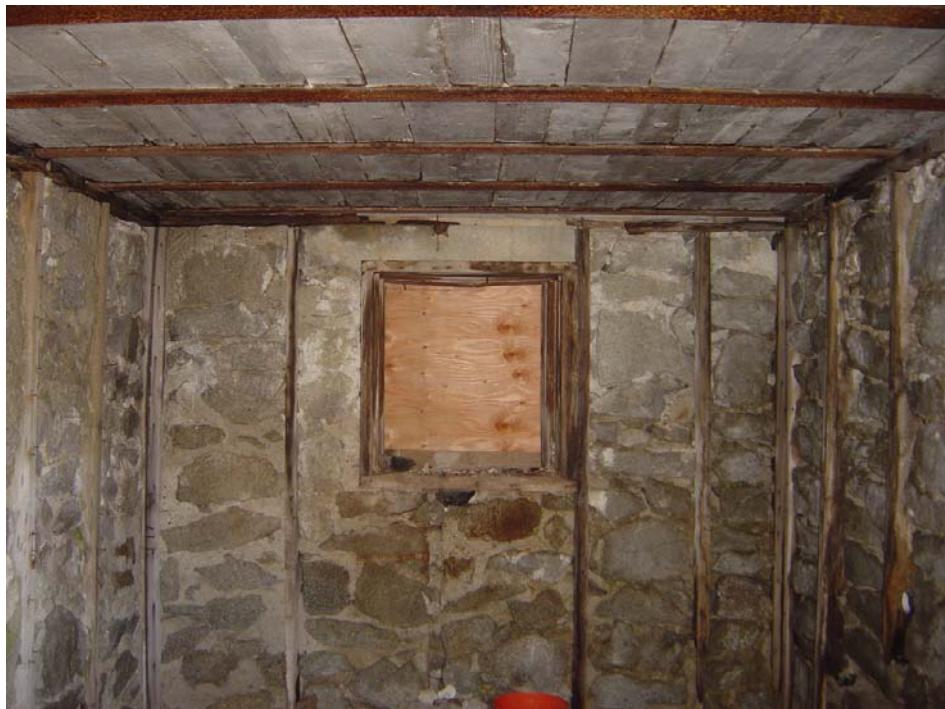
Stewart Irrigation Diversion Building - Building #2451
