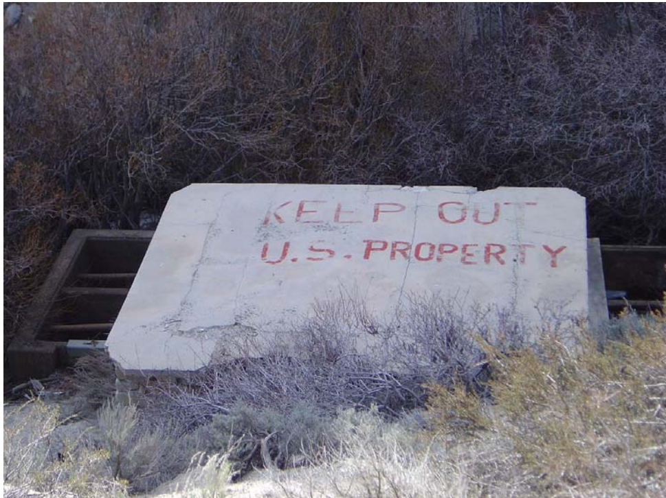
Stewart Irrigation Diversion Building - Building #2451
