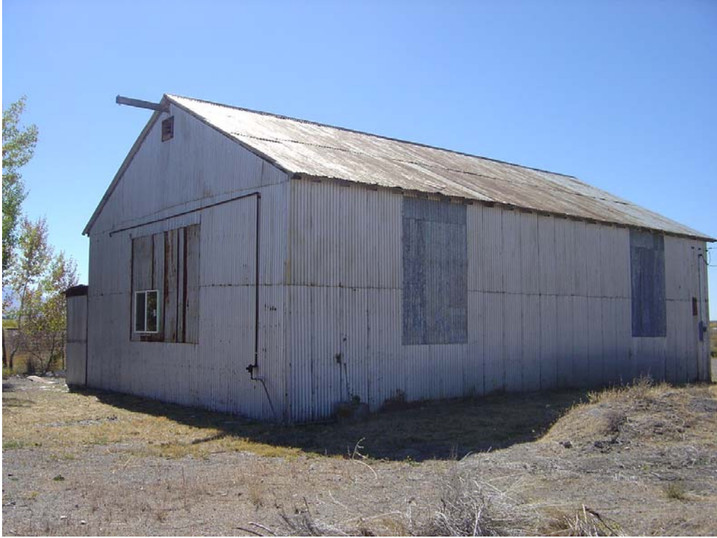
NDF Volunteer Fire Station - Building #0600 Description: Exterior view of the building.
