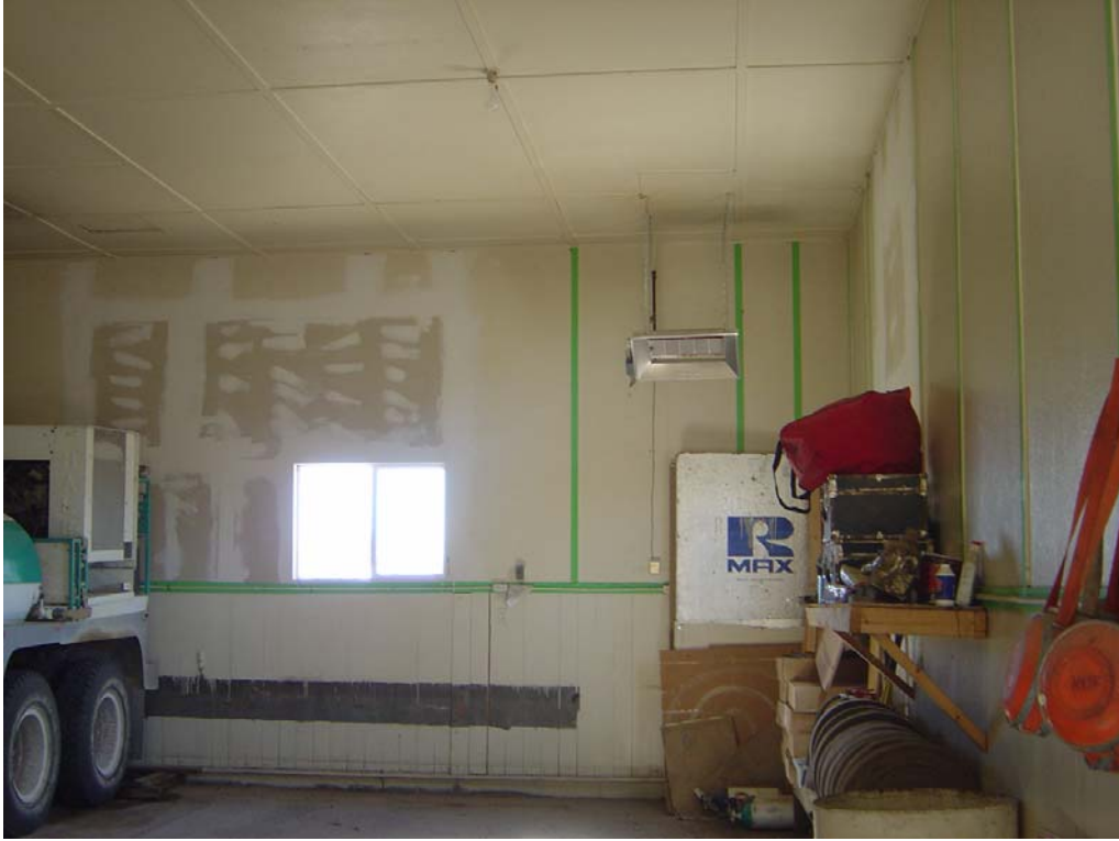
NDF Volunteer Fire Station - Building #0600 Description: Interior of building.
