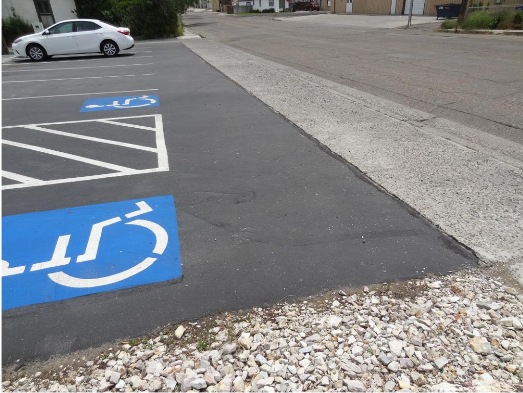
Elko DETR - Site #9823 Description: Craft fill and seal of asphalt paving needed.
