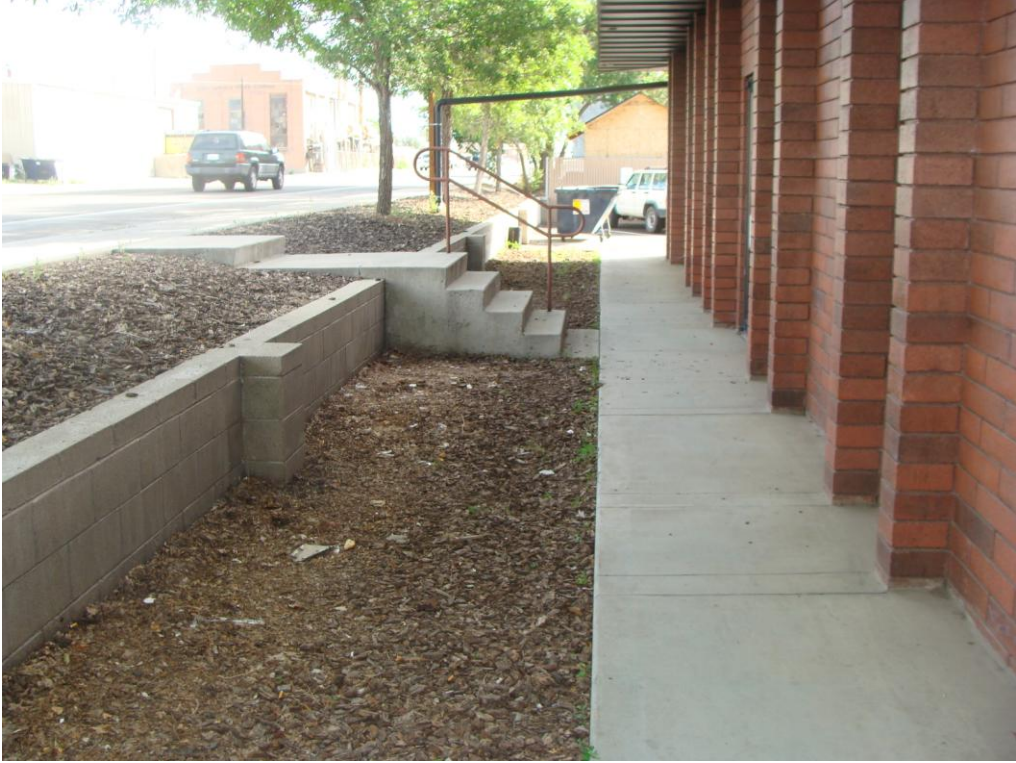
DETR Elko Office - Site #9823 Description: Stairs in need of handrails.
