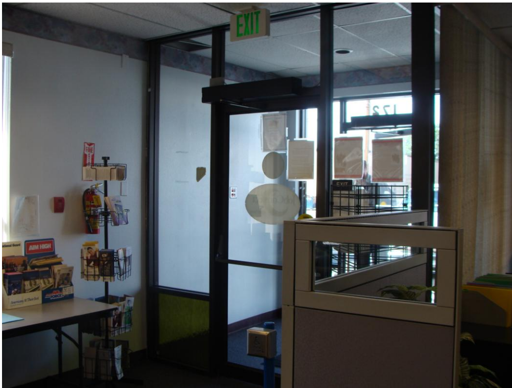
DETR Elko Office – Building #1476 Description: Entry vestibule.
