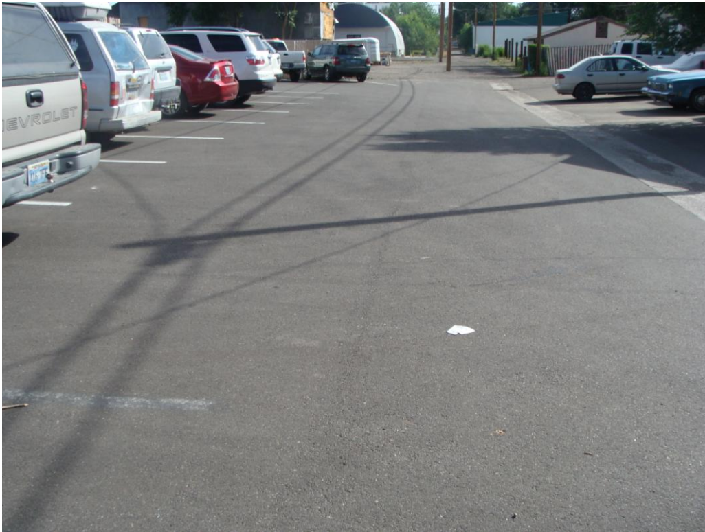
DETR Elko Office - Site #9823 Description: Paved parking area.
