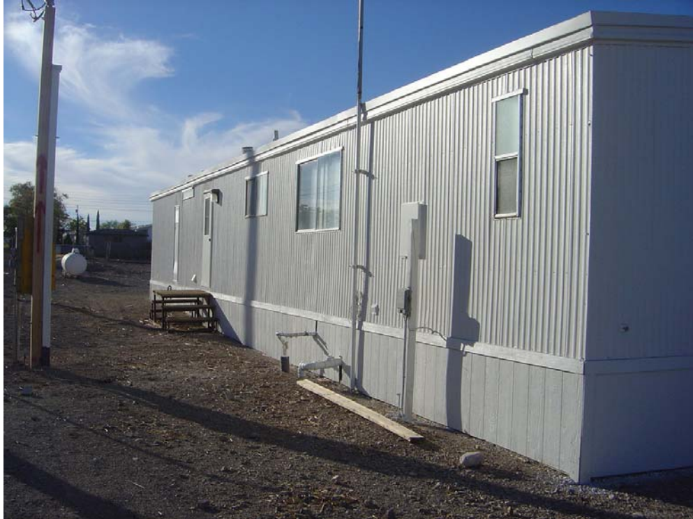
Indian Springs NHP Substation - Building #2462 Description: Exterior view of the building.
