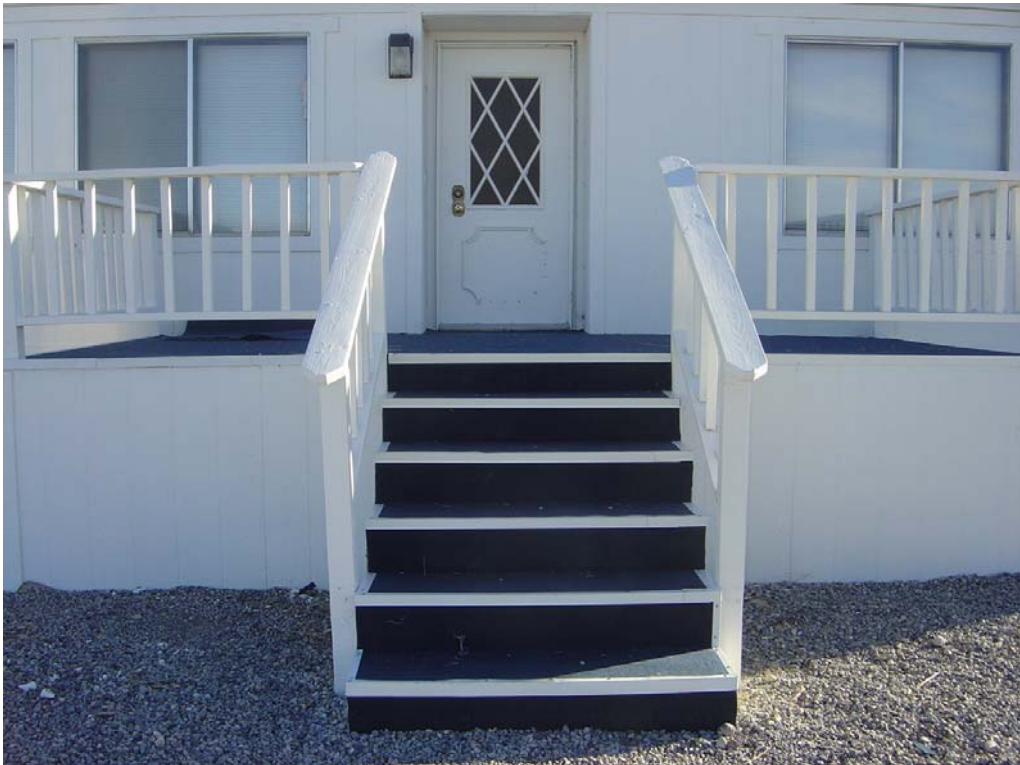
Indian Springs NHP Substation - Building #2462 Description: Entrance into the building.
