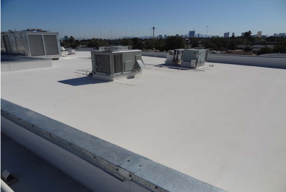
Belrose Office Building - Building #0286 Description: View of the roof and equipment.
