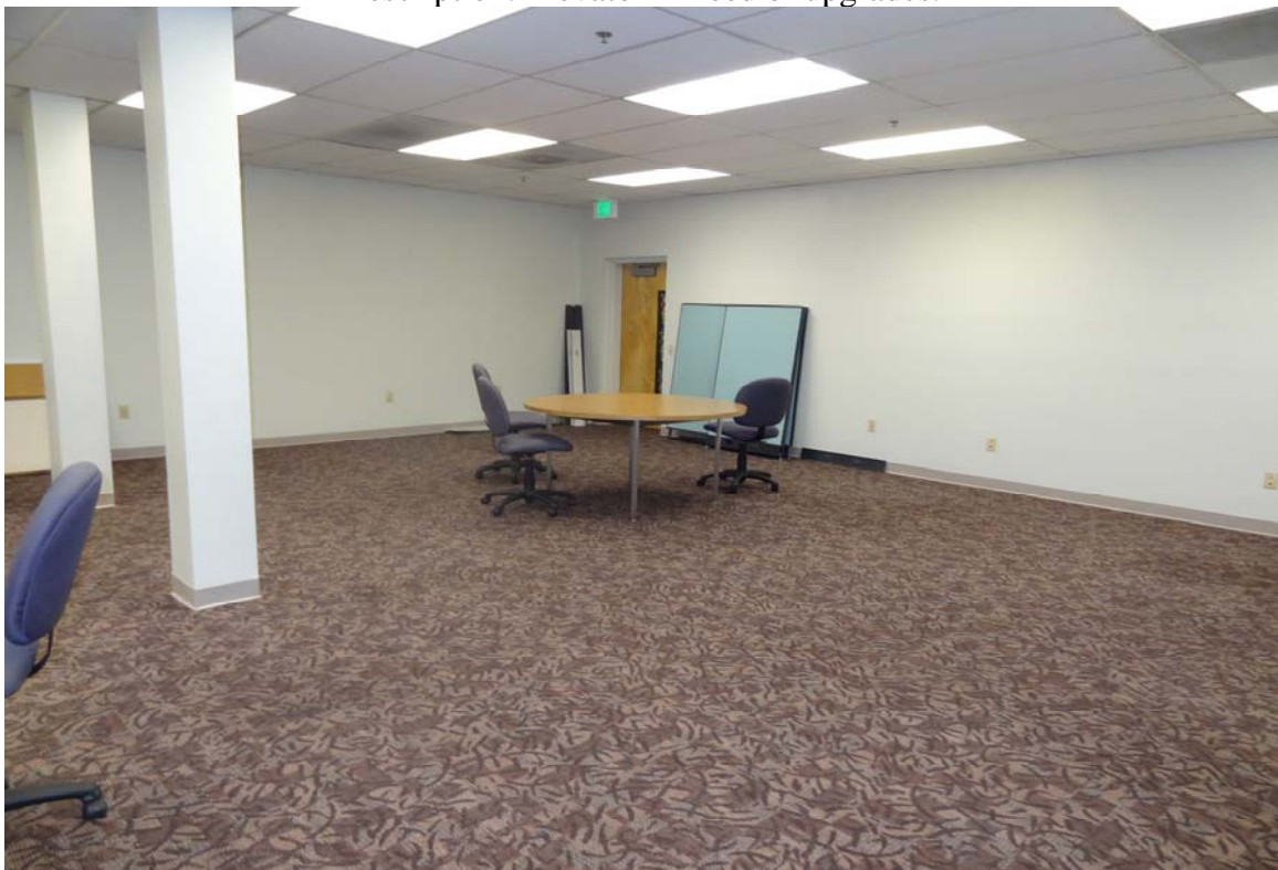
Belrose Office Building - Building #0286 Description: Typical interior office space.
