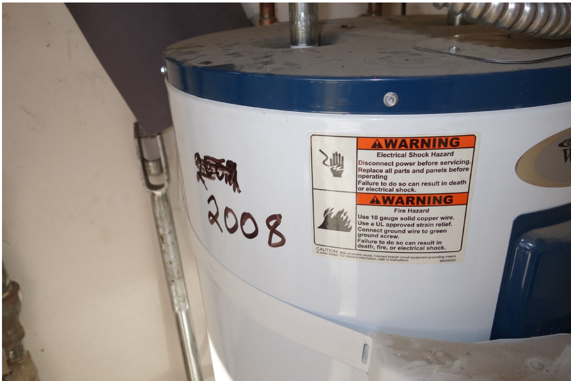
DMV Express Office - Building #0265 Description: Water Heater Replacement Recommended.
