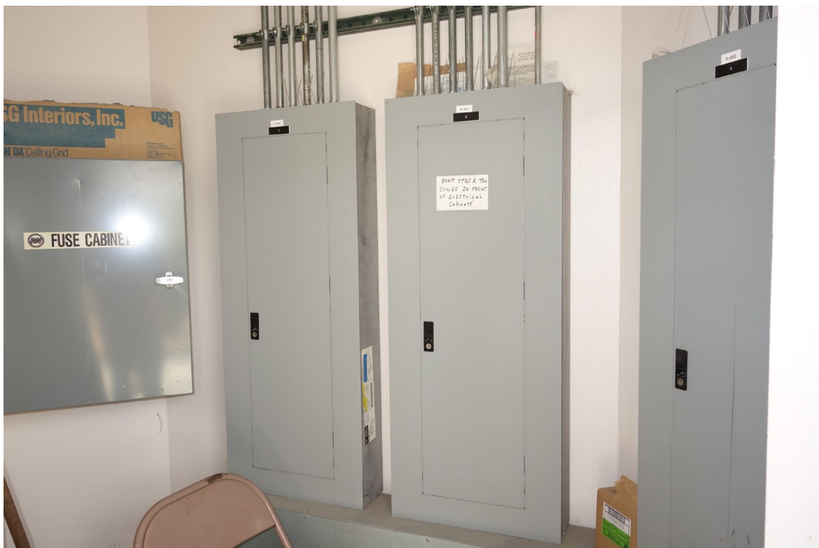
DMV Express Office - Building #0265 Description: Arc Flash Labeling Needed.
