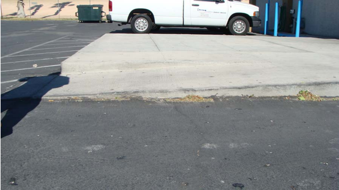
Las Vegas Casual Labor Office Site - Site #9833 Description: ADA accessible ramp.
