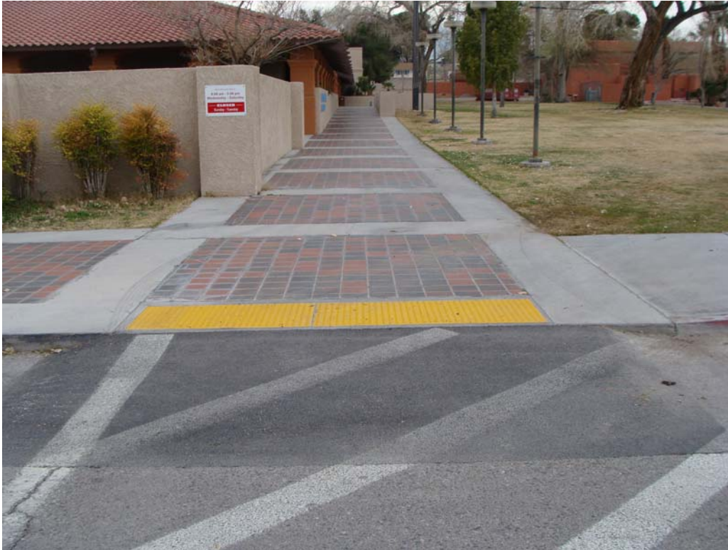
Las Vegas Museum & Historical Society Site - Site #9834 Description: Accessible route of travel from parking to entrance.
