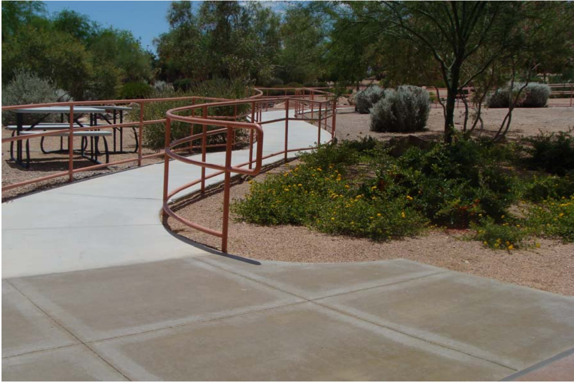
Grant Sawyer Office Site - Site #9835 Description: View of the site walkways.
