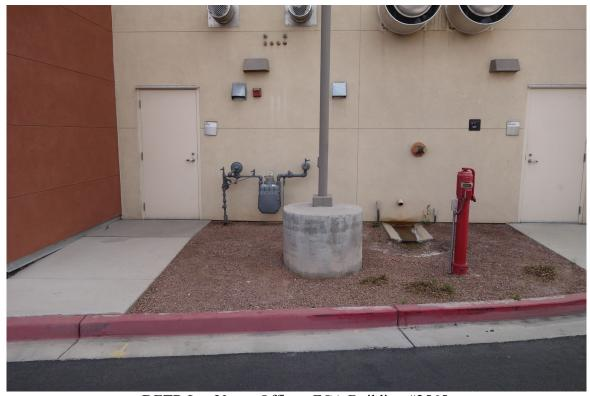
DETR Las Vegas Office - FCA Building #2565 Description: Seismic Gas Isolation Valve Needed.
