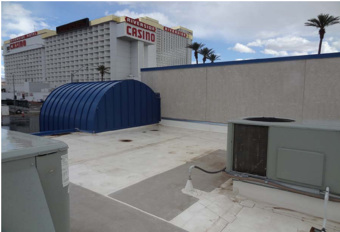
Laughlin Wildlife Field Office - Building #2470 Description: View of the roof & equipment.
