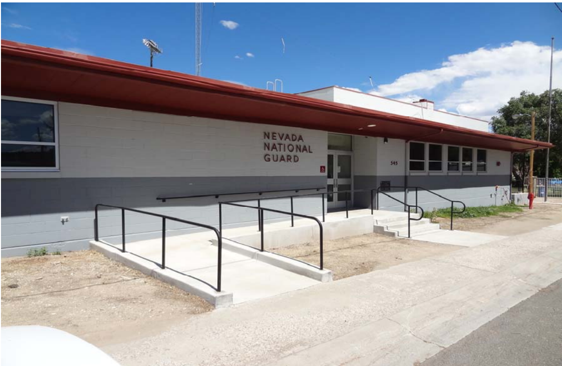
Ely Armory - Building #0676 Description: ADA accessible ramp into building.
