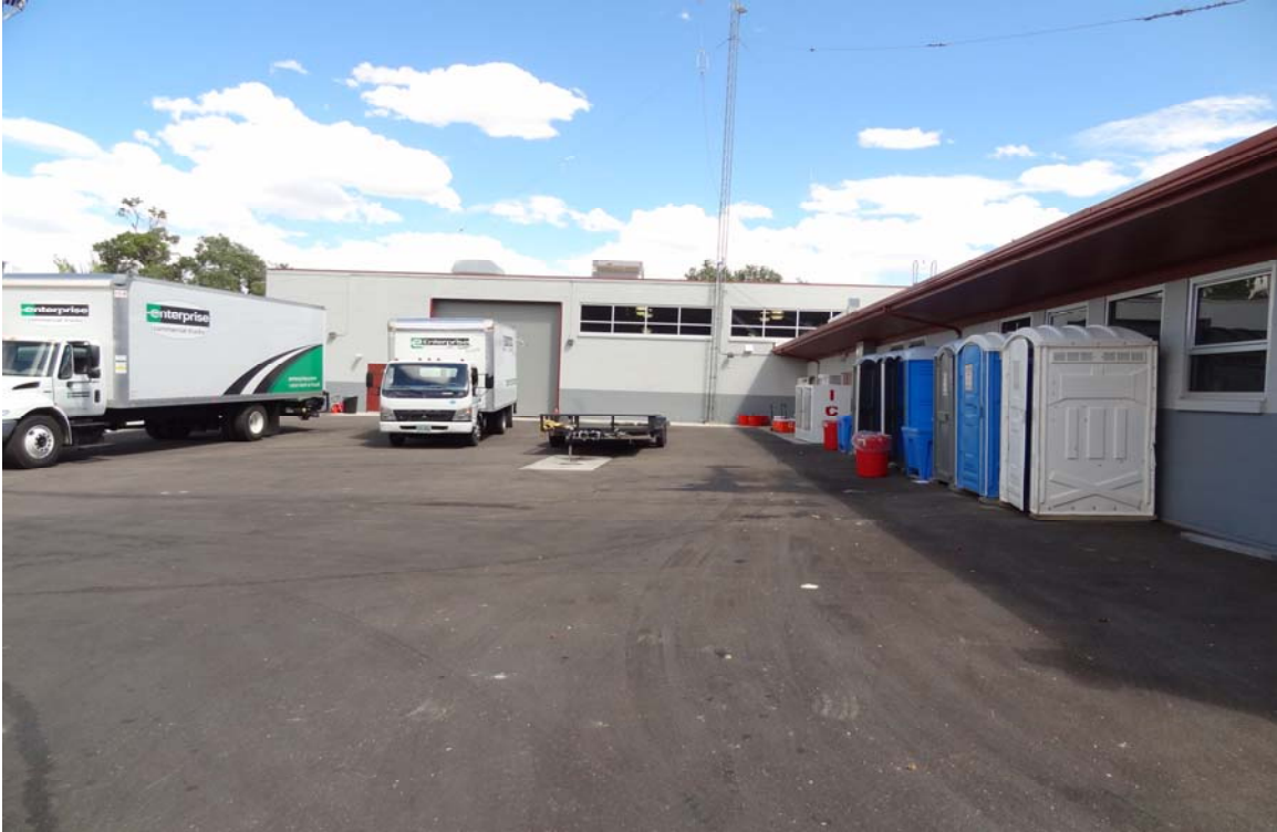
Ely Armory Site - Site #9841 Description: AC paving on north side of the building.
