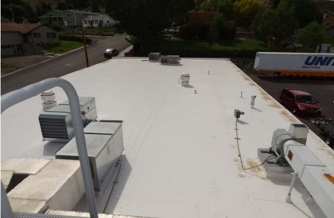
Ely Armory - Building #0676 Description: View of the roof and equipment.
