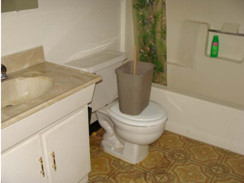
Lee Canyon Fire Station No. 2 - Building #0284 Description: Interior of the restroom.
