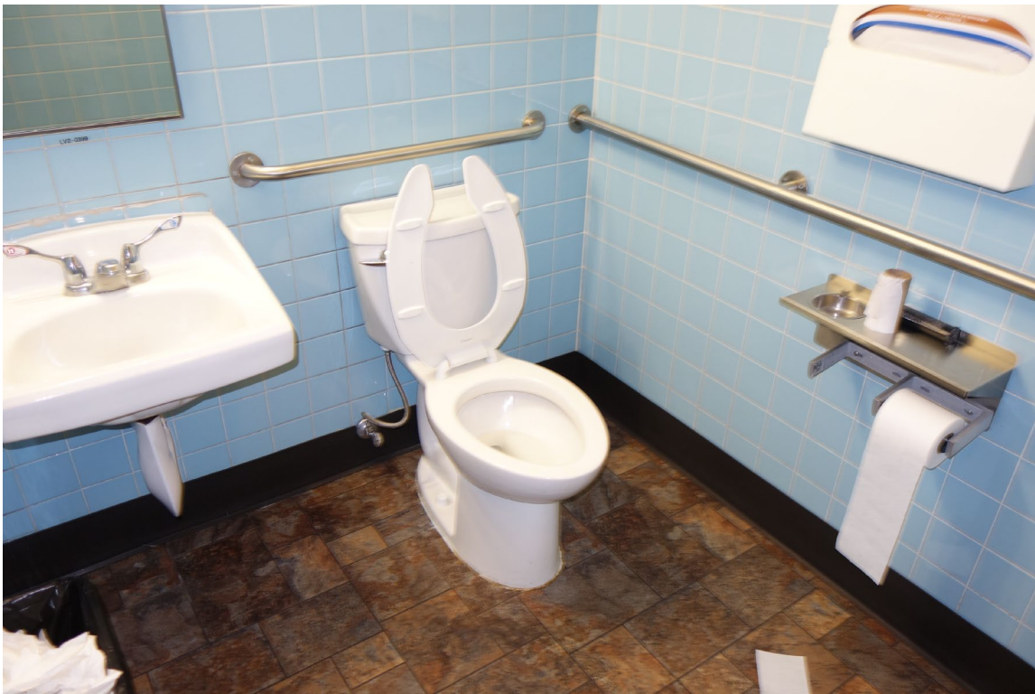
Reno Purchasing Warehouse - Building #0399 Description: View of Non-ADA Compliant Restroom - Toilet too far from wall.
