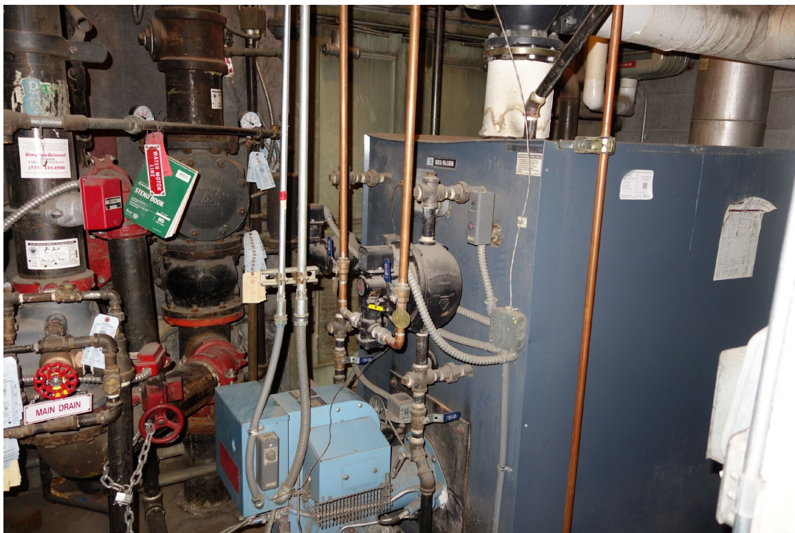
Reno Purchasing Warehouse - Building #0399 Description: Boiler Replacement Planning Recommended.
