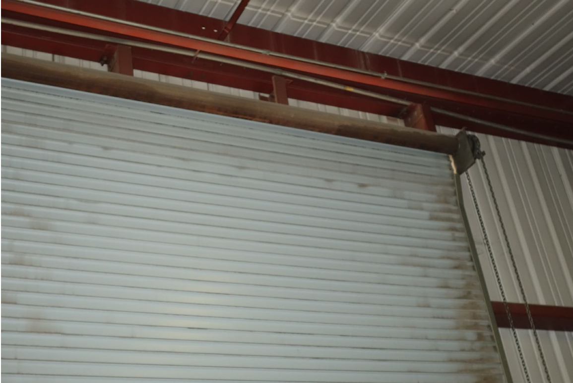
Storage Building - Building #3098 Description: Overhead Coiling Door Replacement Recommended.
