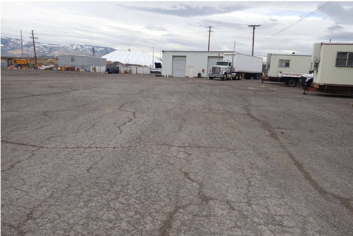
Reno Purchasing Warehouse Site - Site #9845 Description: Damaged AC Paving Replacement Needed.
