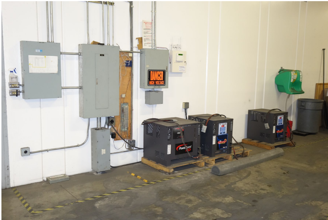
Reno Purchasing Warehouse - Building #0399 Description: Arc Flash Study / Labeling Needed.
