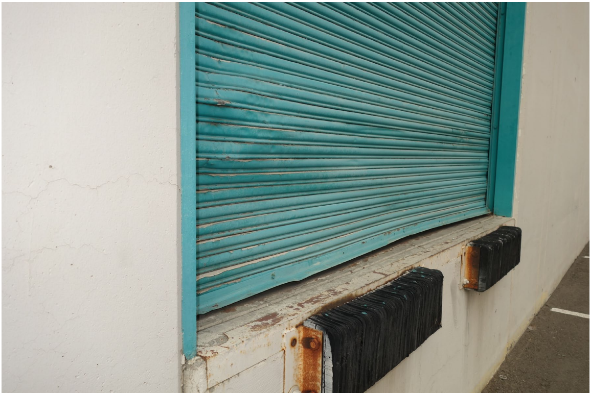
Reno Purchasing Warehouse - Building #0399 Description: Damaged Overhead Coiling Doors Replacement Needed.
