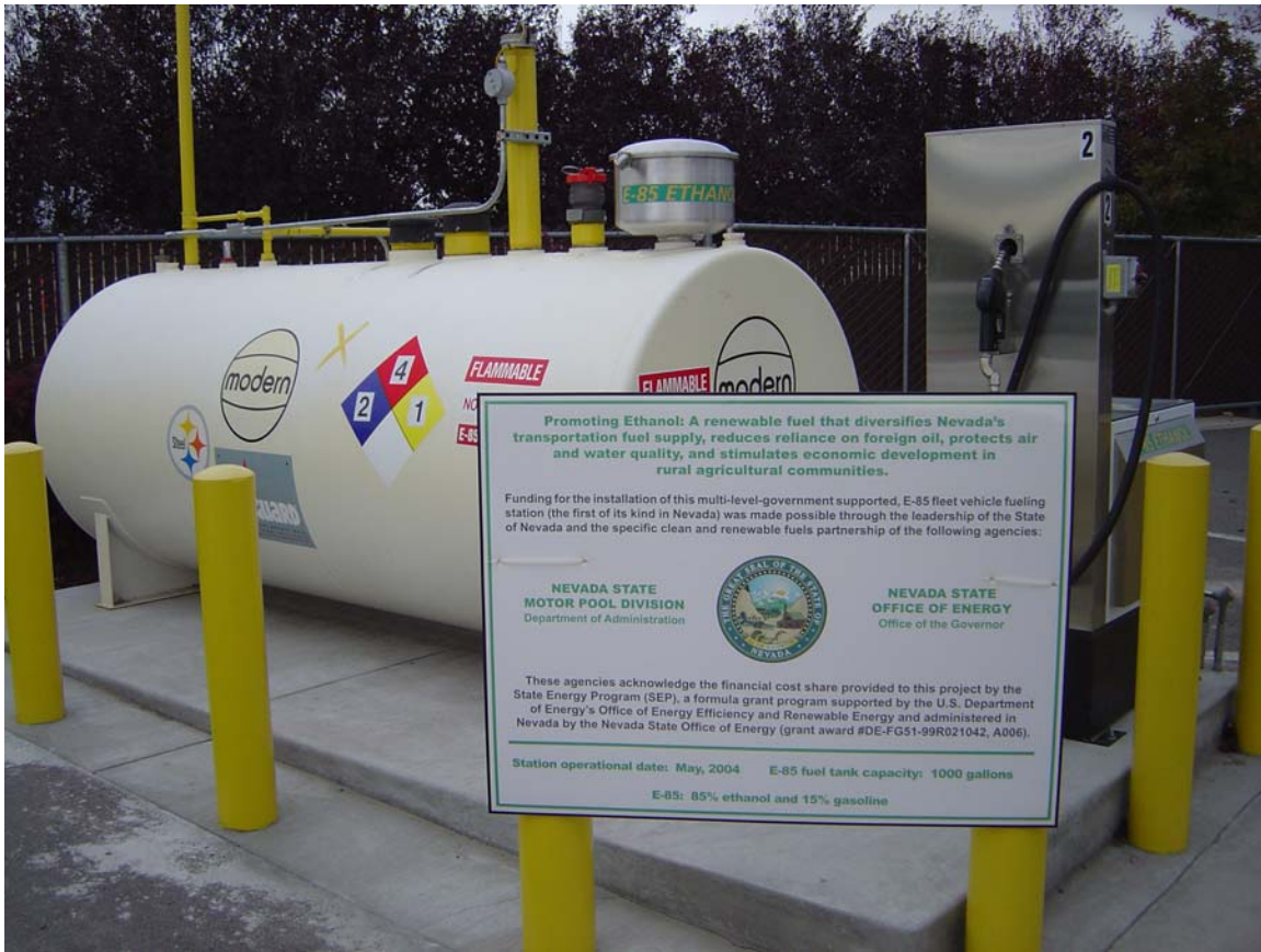
Reno Motor Pool Index No. 2483 Description: Ethanol fueling station.
