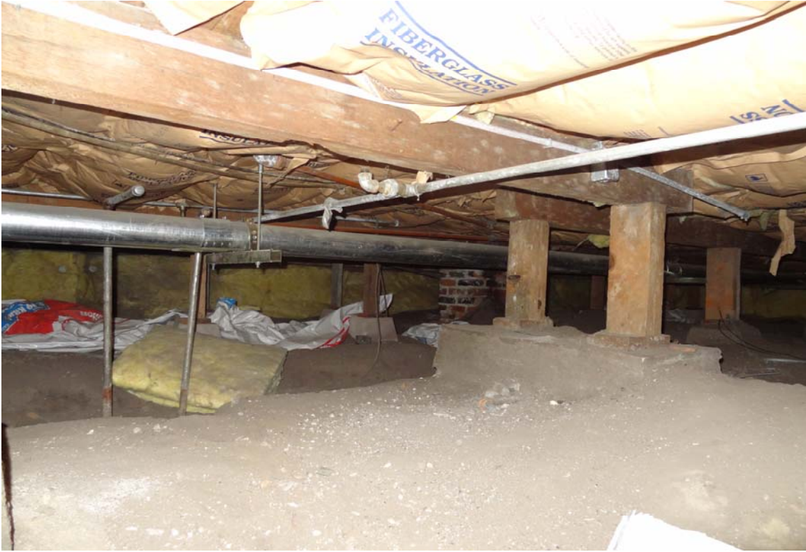
Museum Administration Office - Building #2028 Description: Crawl space / basement.
