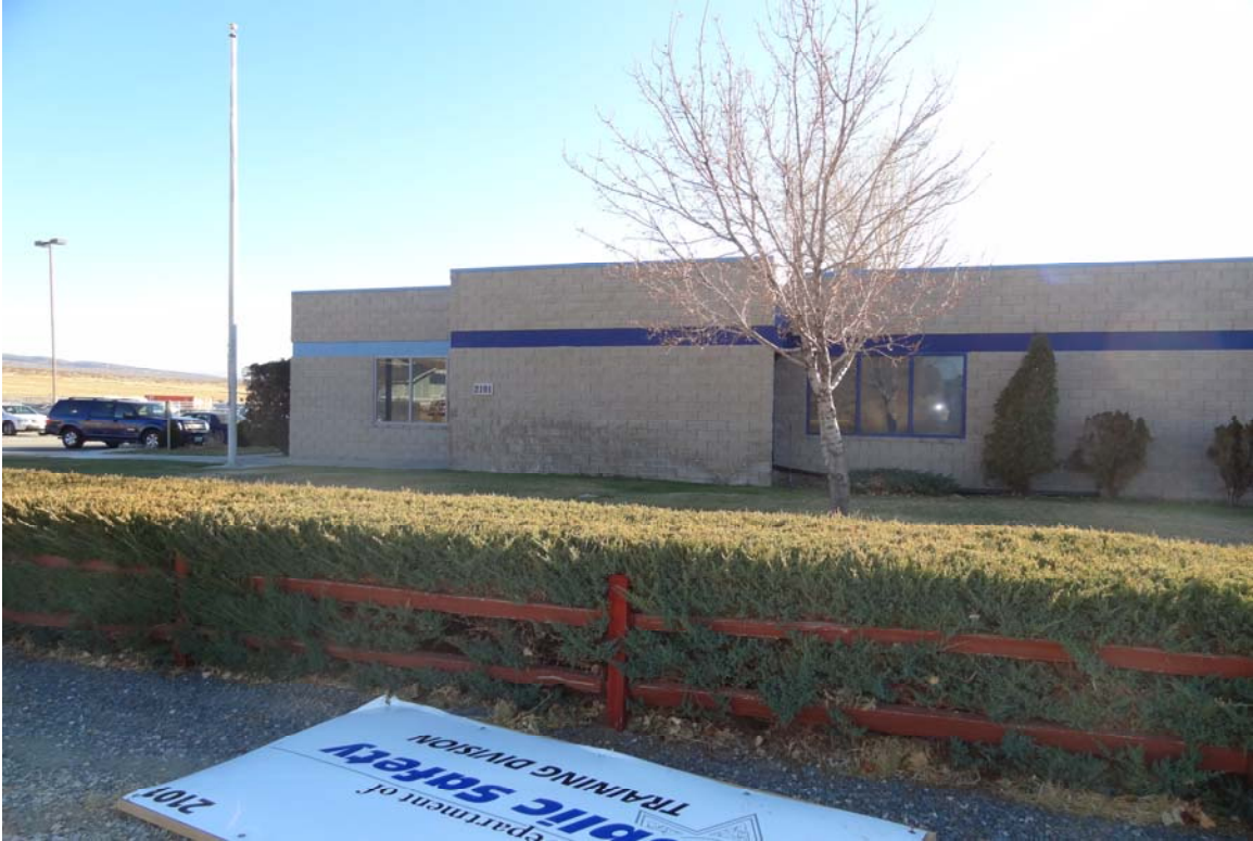
DPS Training Facility - Building #0898 Description: Exterior of the building.
