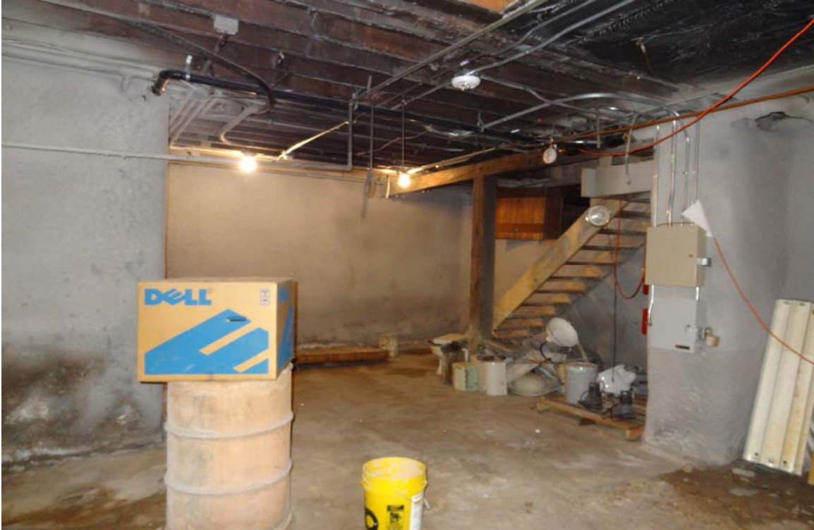
East Ely Railroad Depot - Building #2227 Description: View of the basement.
