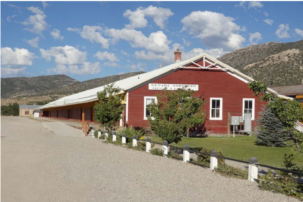
East Ely Railroad Freight Barn - Building #2128 Description: Exterior of the building.
