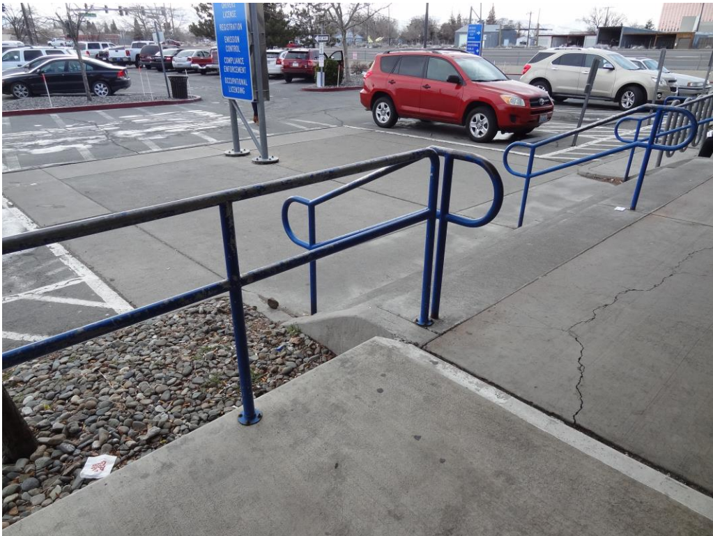
Reno DMV Site - Site #9858 Description: Cracked concrete and asphalt at entrance.
