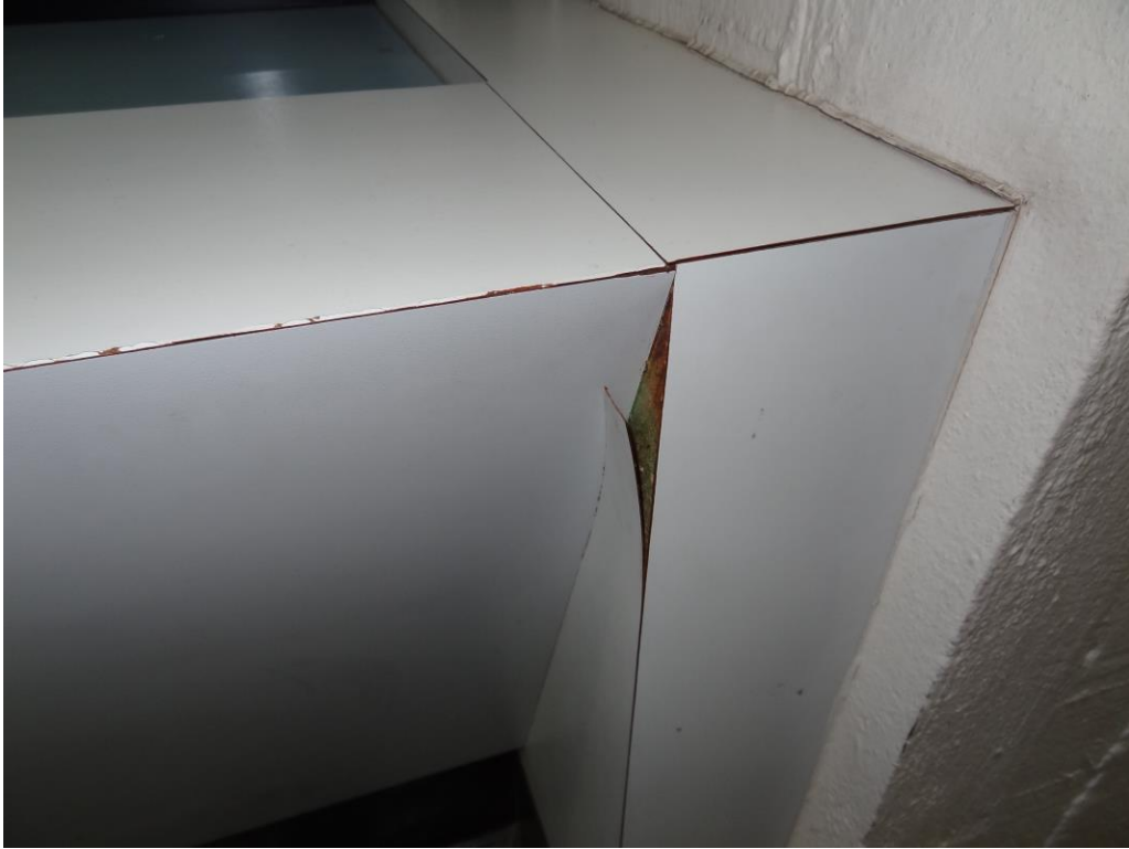
DMV Reno Office - Building #0272 Description: Typical damaged casework at customer stations.
