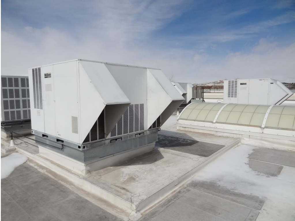
DMV Reno Office - Building #0272 Description: 23 year old rooftop HVAC equipment.
