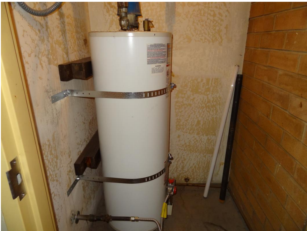
DMV Reno Office - Building #0272 Description: 21 year old water heater.
