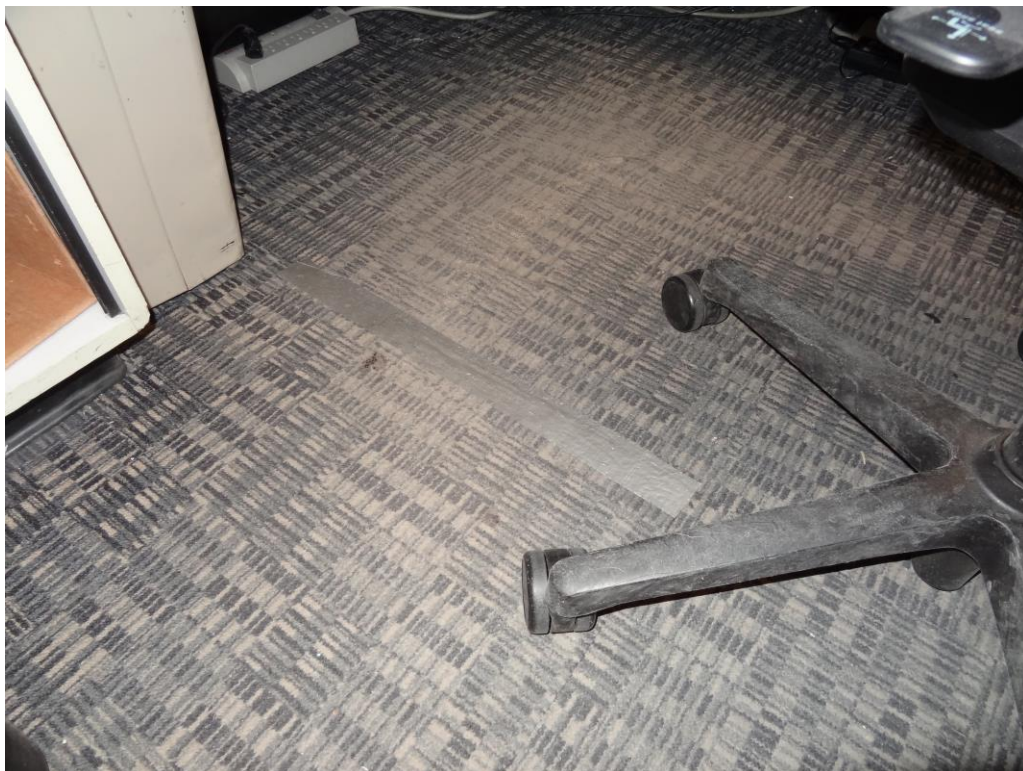
DMV Reno Office - Building #0272 Description: Carpet repaired with duct tape and due for replacement.
