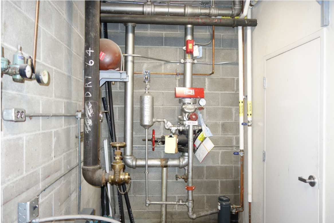
Blasdel Office Building - Building #0200 Description: Fire Sprinkler Riser in Basement.
