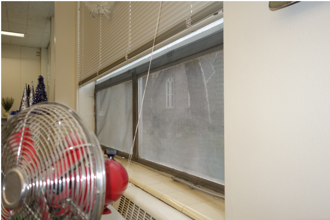
Blasdel Office Building - Building #0200 Description: Window & Hydronic Baseboard Replacement Needed.
