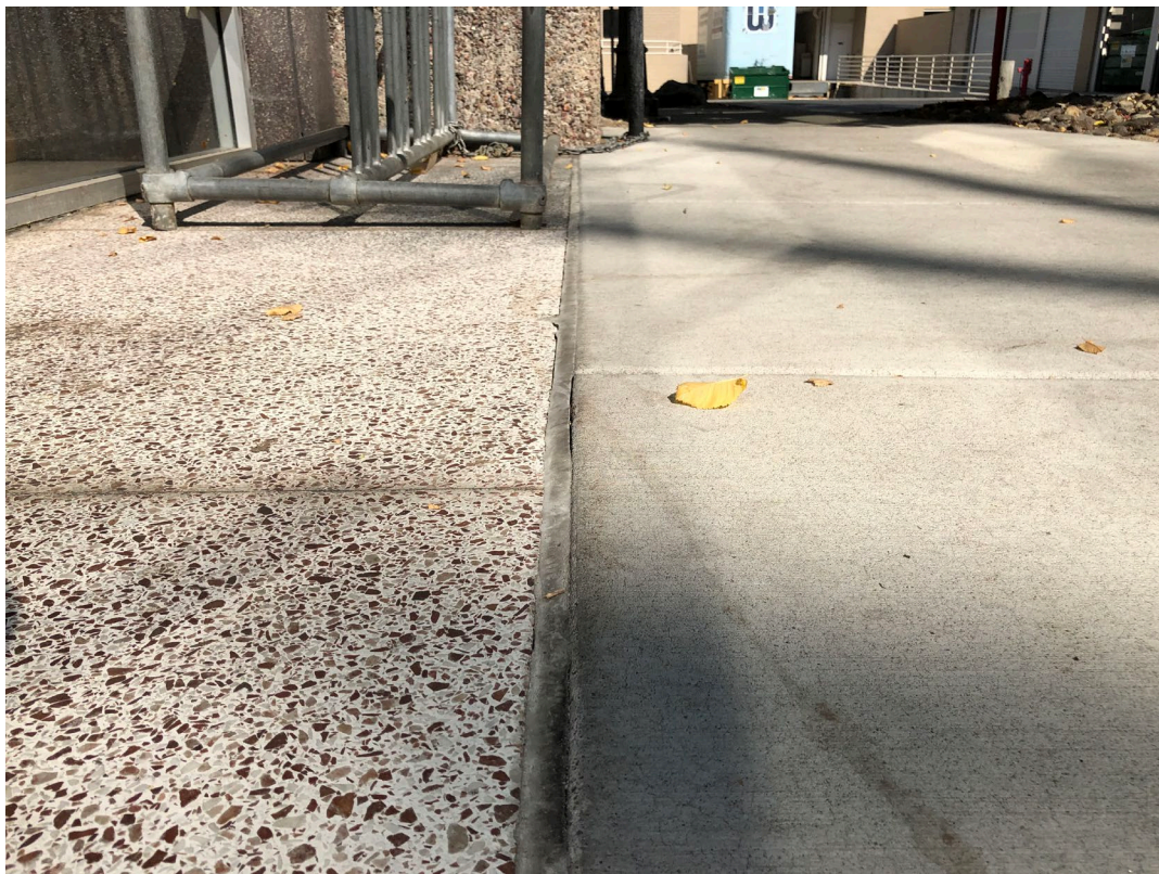
Blasdel Office Building - Building #0200 Description: Walking Surface Creating Ponding Water at South Entrance.
