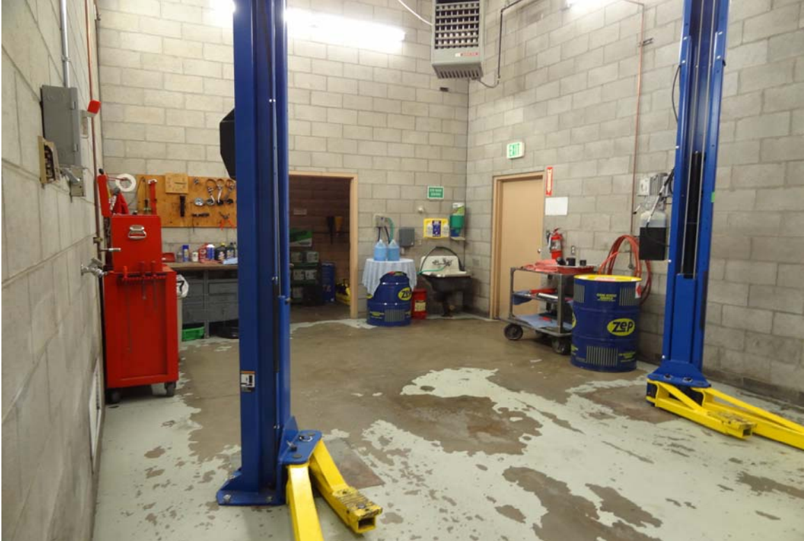
Carson City Motor Pool - Building #0204 Description: View of the repair bay.
