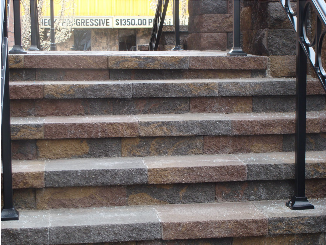
Paul Laxalt State Building Site - Site #9863 Description: Laxalt Plaza Stair Modifications – Risers Exceeding 3/8” Variation.
