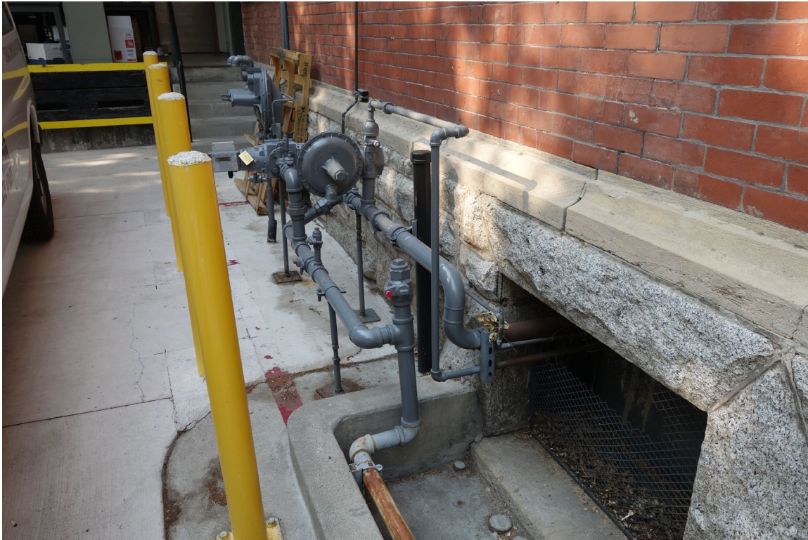
Paul Laxalt State Building – Building #0394 Description: Seismic Gas Shut-off Valve Needed.
