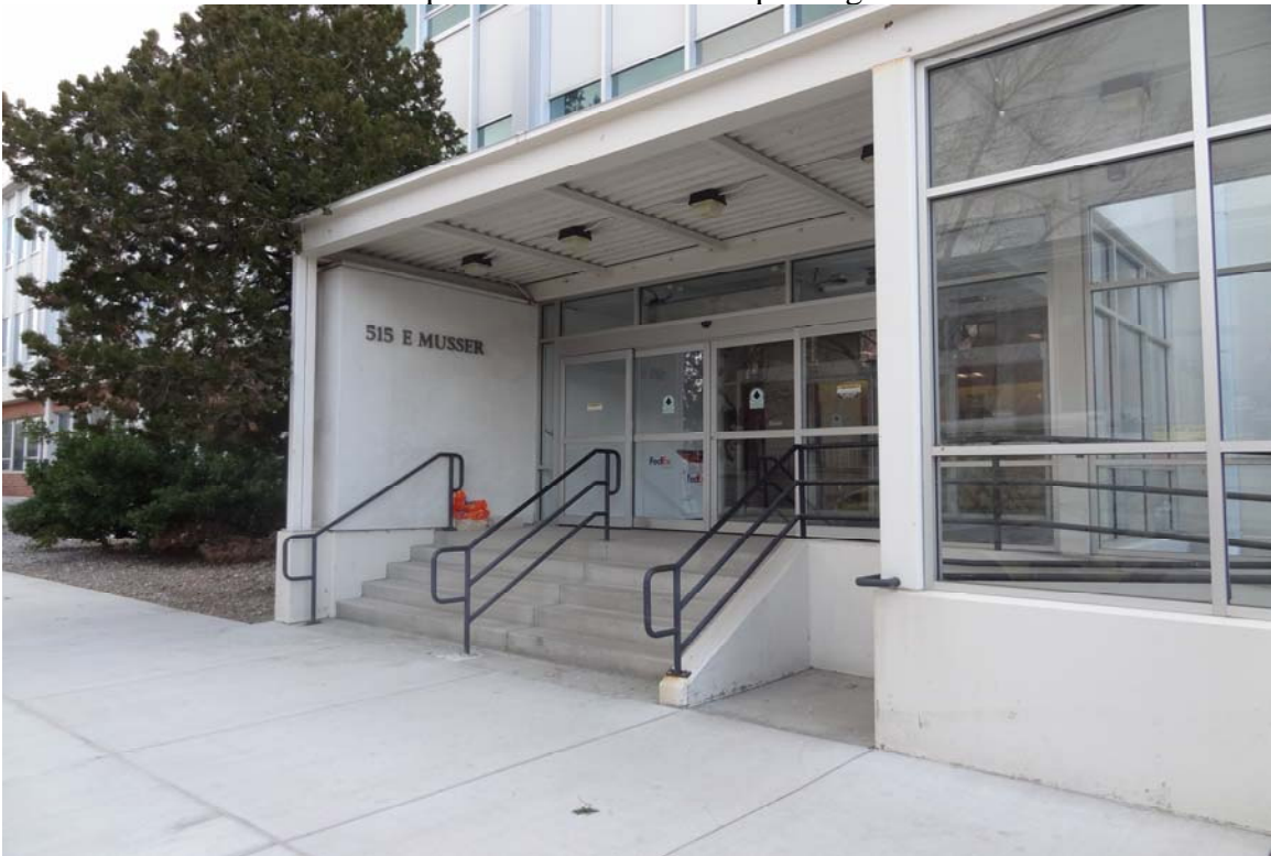
Carson City State Offices - Building #0397 Description: Public entrance.
