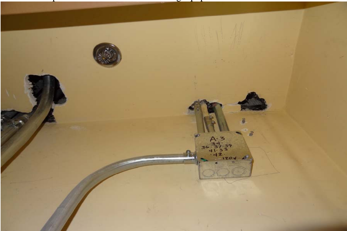
Carson City State Offices - Building #0397
