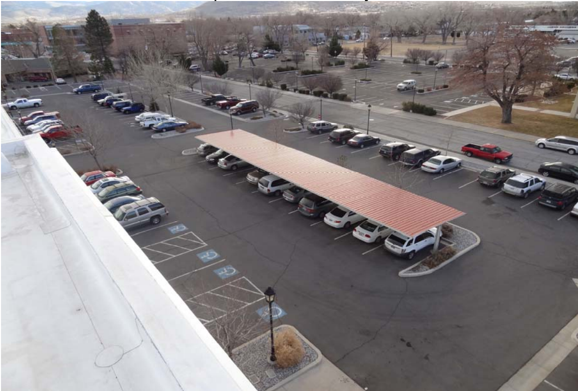
State Offices Carport - Building #3110
