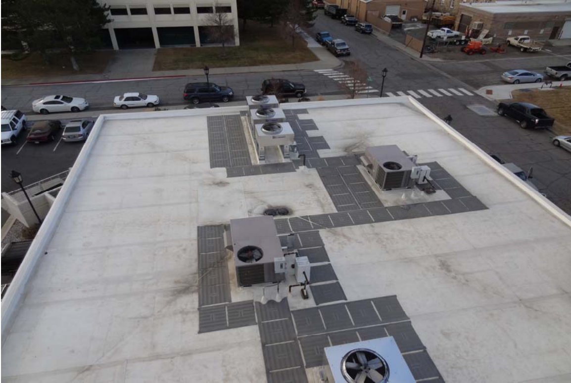
Carson City State Offices - Building #0397
