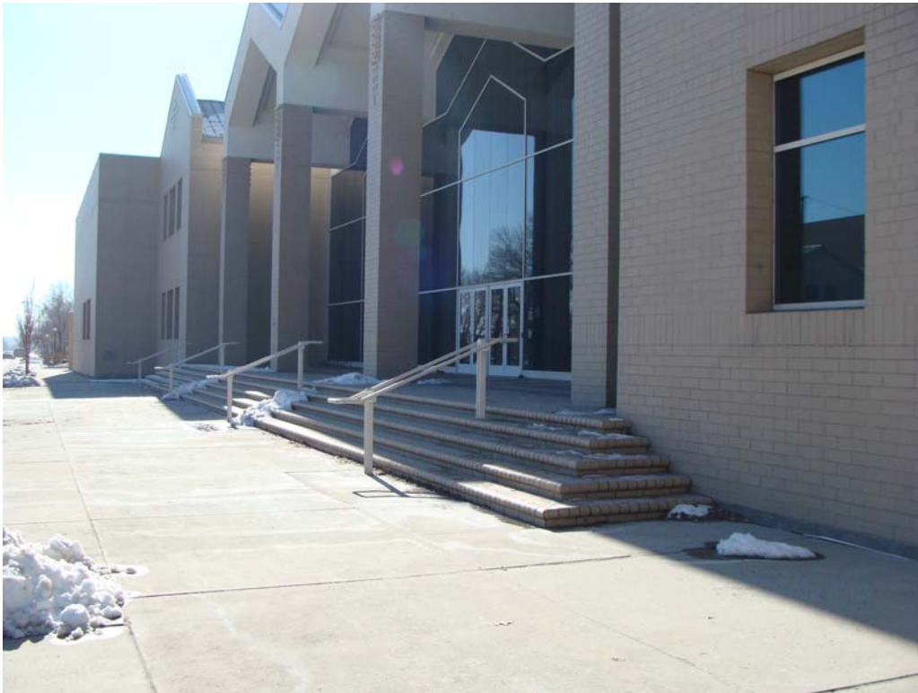
Nevada State Library & Archives - Building #1675 Description: Public entrance off of Stewart Street.
