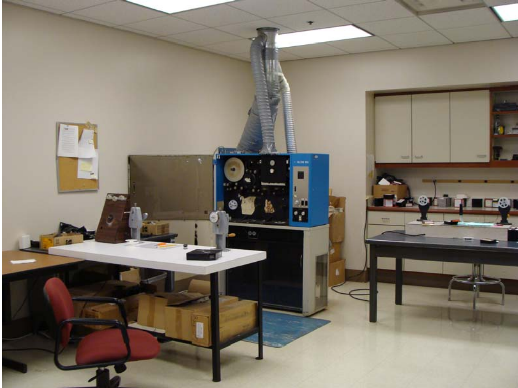
Nevada State Library & Archives - Building #1675 Description: Ammonia processing machine in need of venting modifications.
