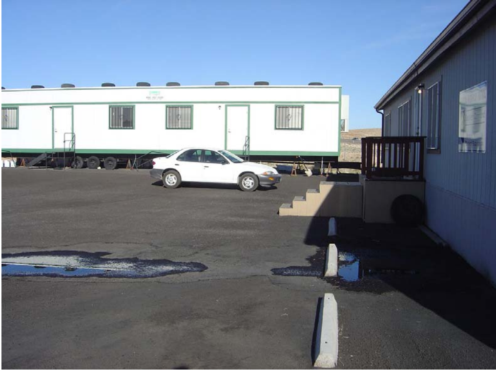
Moapa/Mesquite NHP Substation – Site # 9873 Description: Site looking east.
