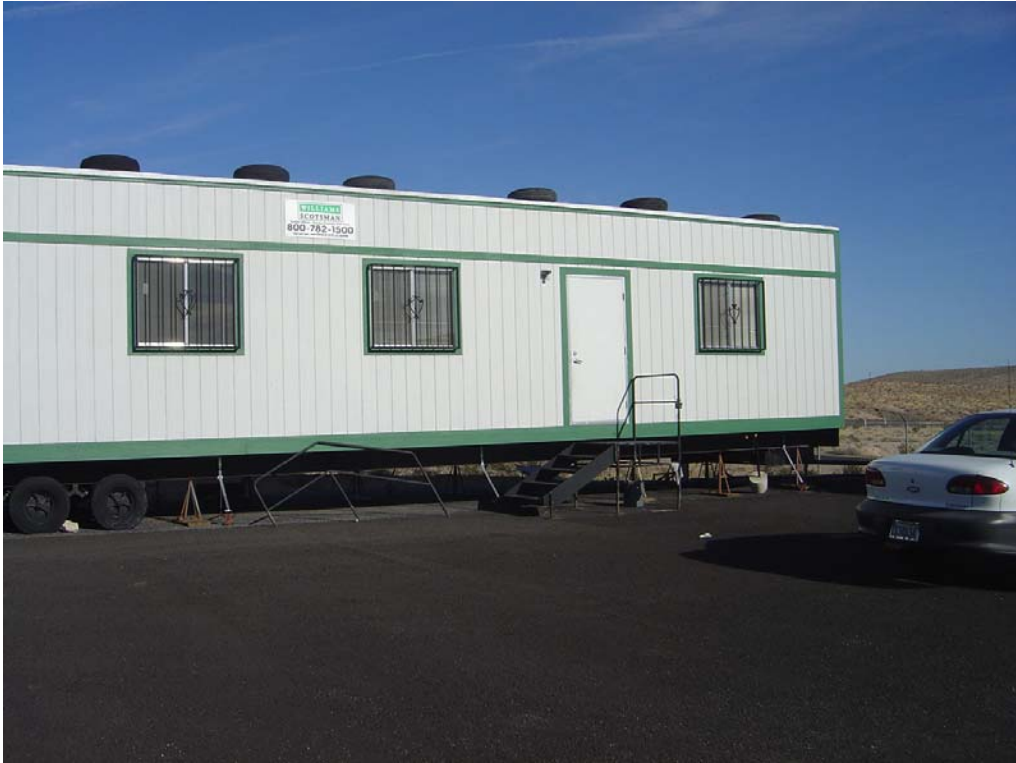
Moapa/Mesquite NHP Substation – Building #2566 Description: Exterior of modular office.
