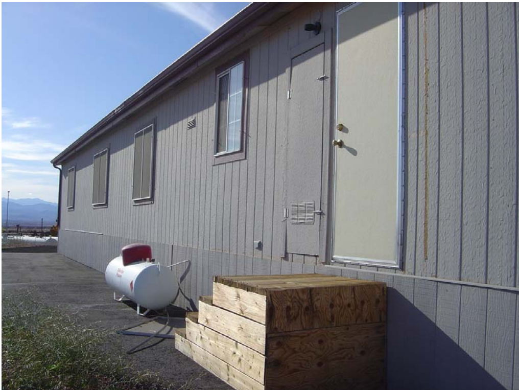
Moapa/Mesquite NHP Substation – Building #2463 Description: Stairs on south side of residence.
