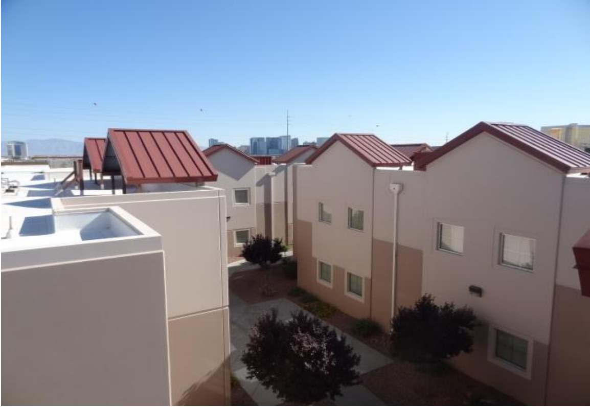
Residential Building B – FCA Building #2560 Description: Exterior of the building.
