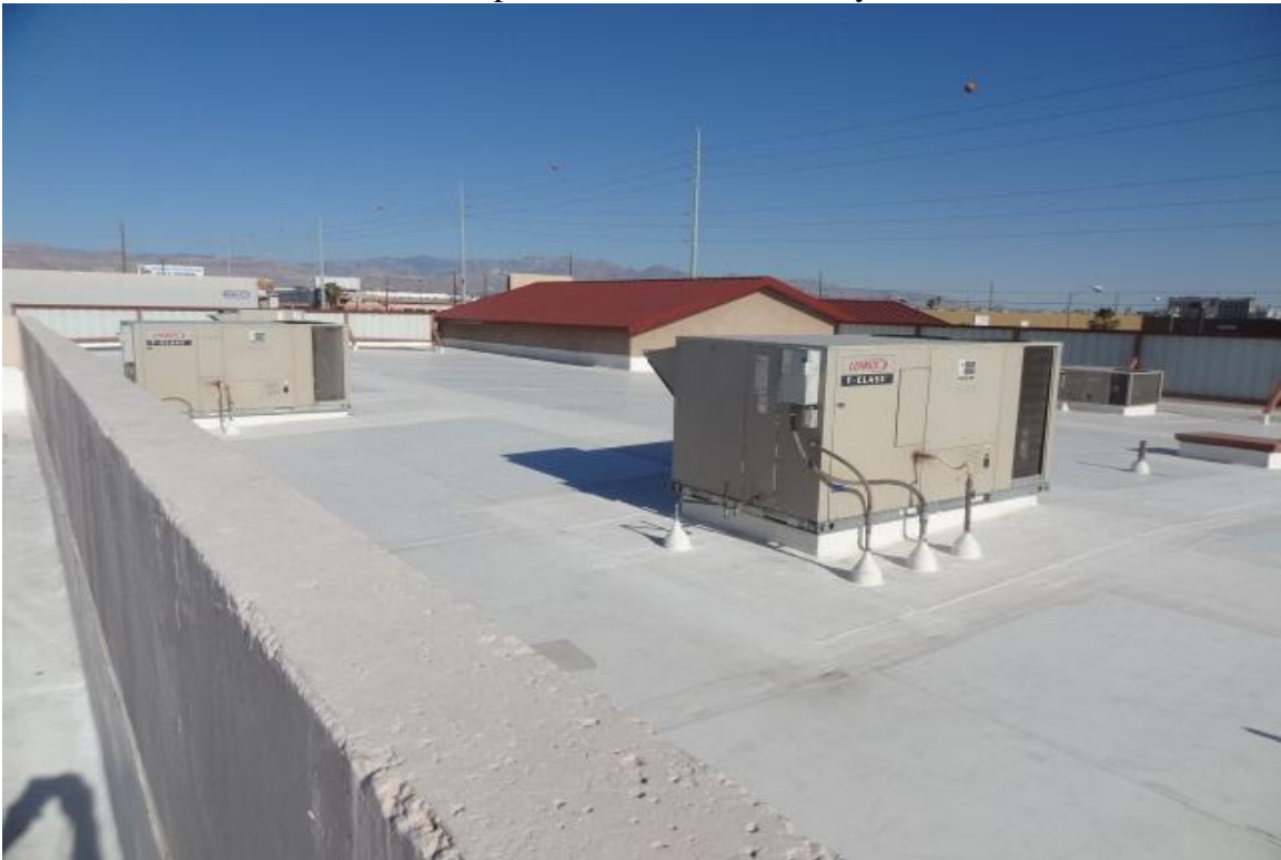
Administration Building – FCA Building #2559 Description: View of the roof / equipment.
