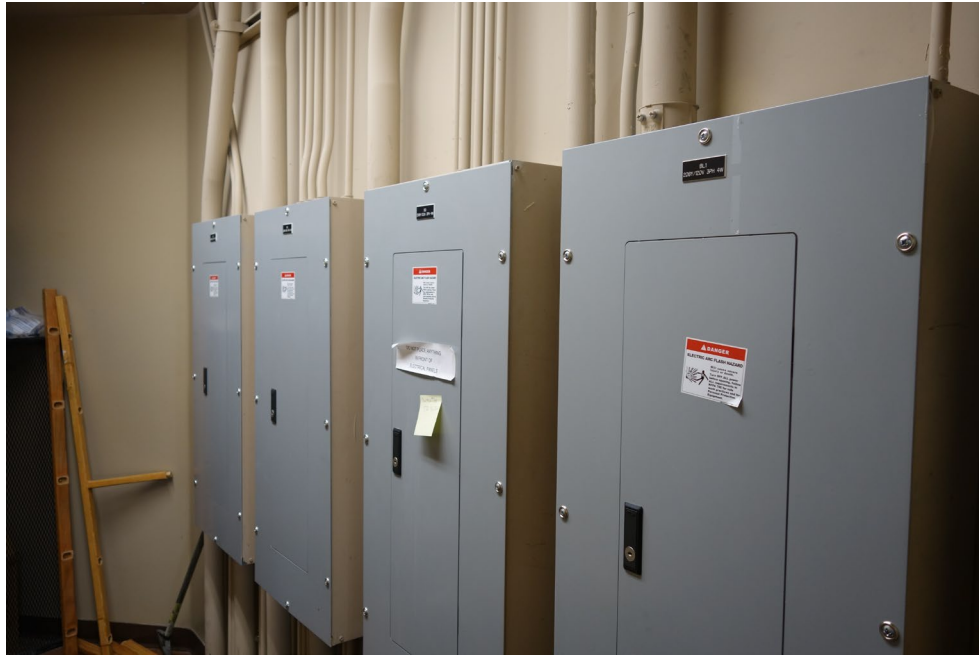
Residential Unit #1 – FCA Building #2560 Description: Arc Flash & Breaker Coordination Study Needed.
