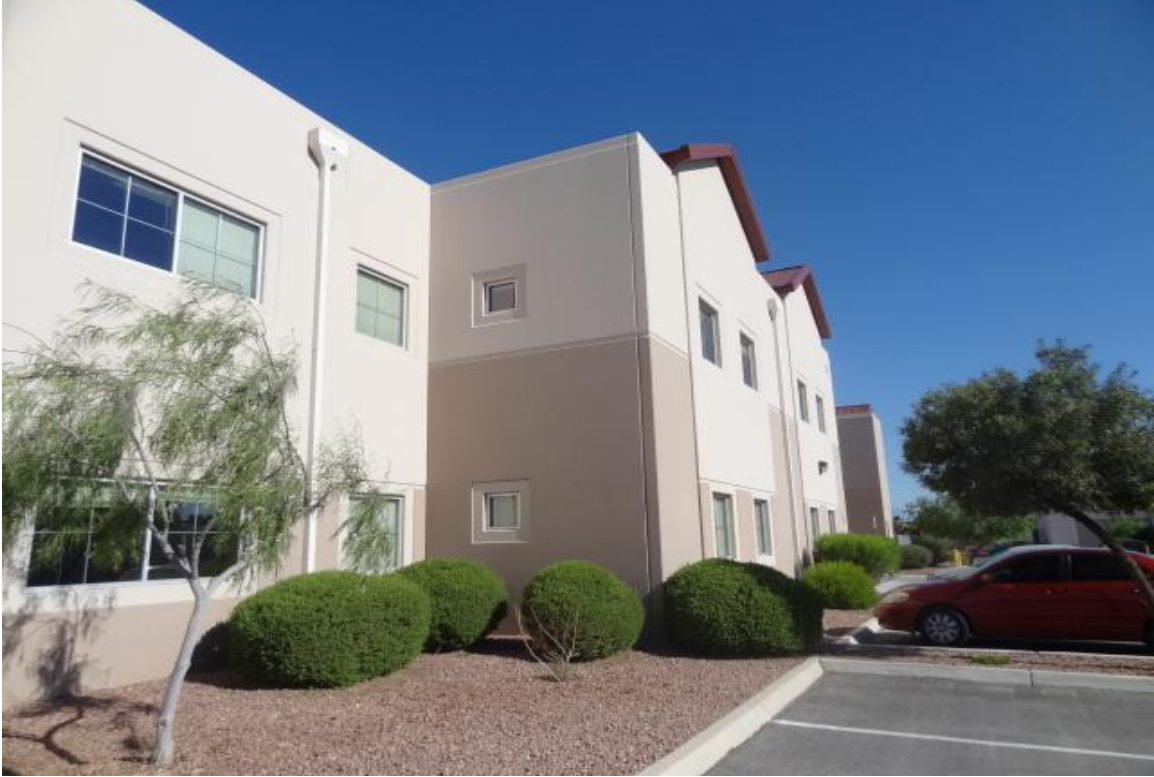
Residential Building C – FCA Building #2561 Description: Exterior of the building.
