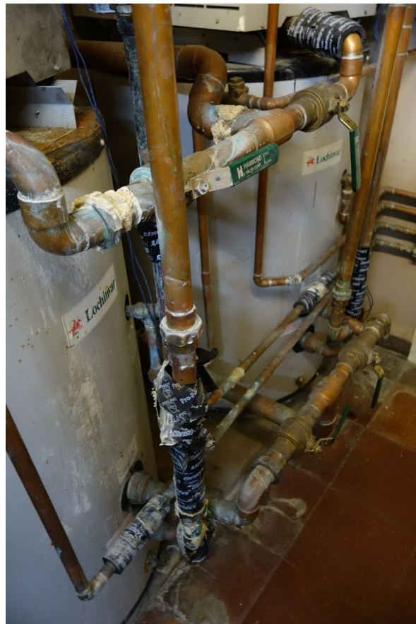
Residential Unit #1 – FCA Building #2560 Description: Boiler Replacement & Water Treatment Needed.
