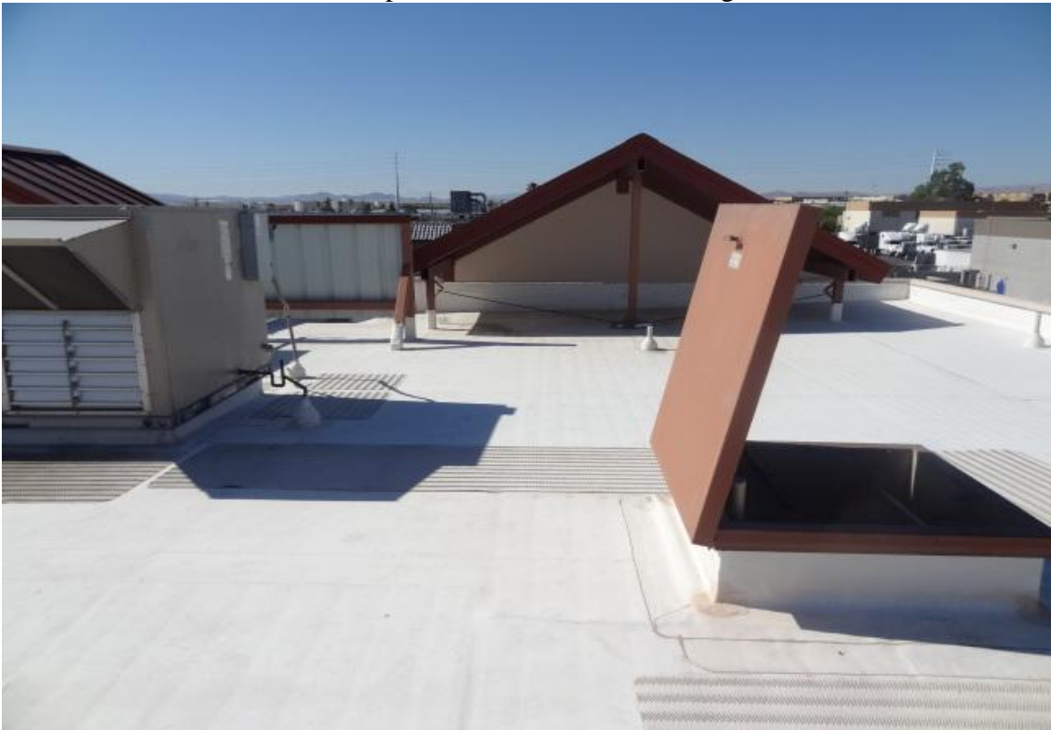
Residential Building C – FCA Building #2561 Description: View of the roof.
