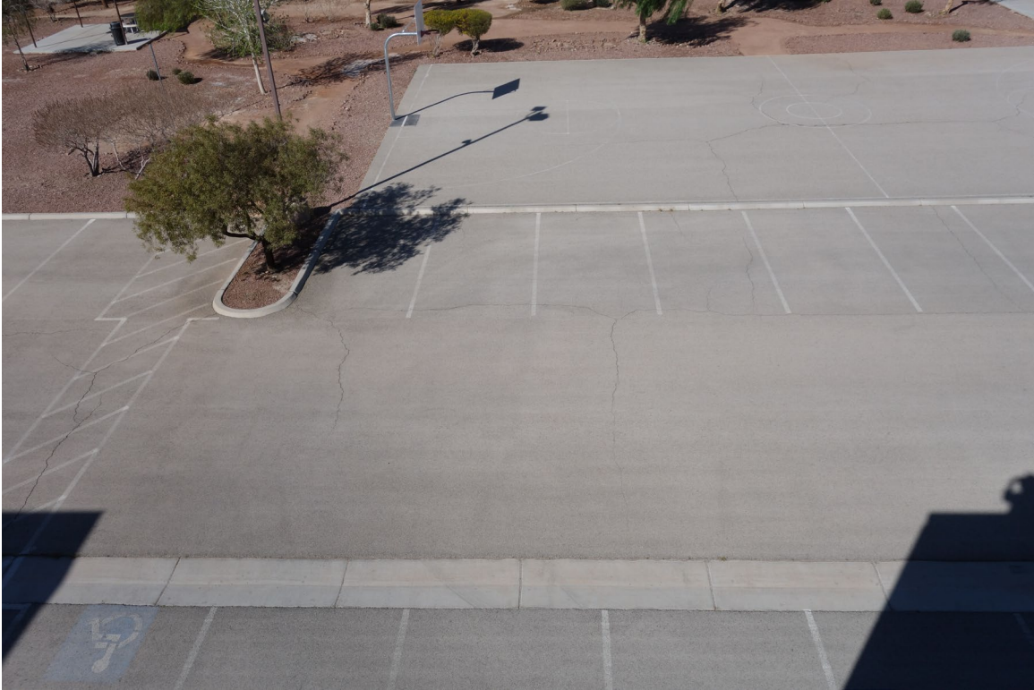
Casa Grande Transitional Center Site – FCA Site #9875 Description: Crack fill / Seal Asphalt Paving Needed.
