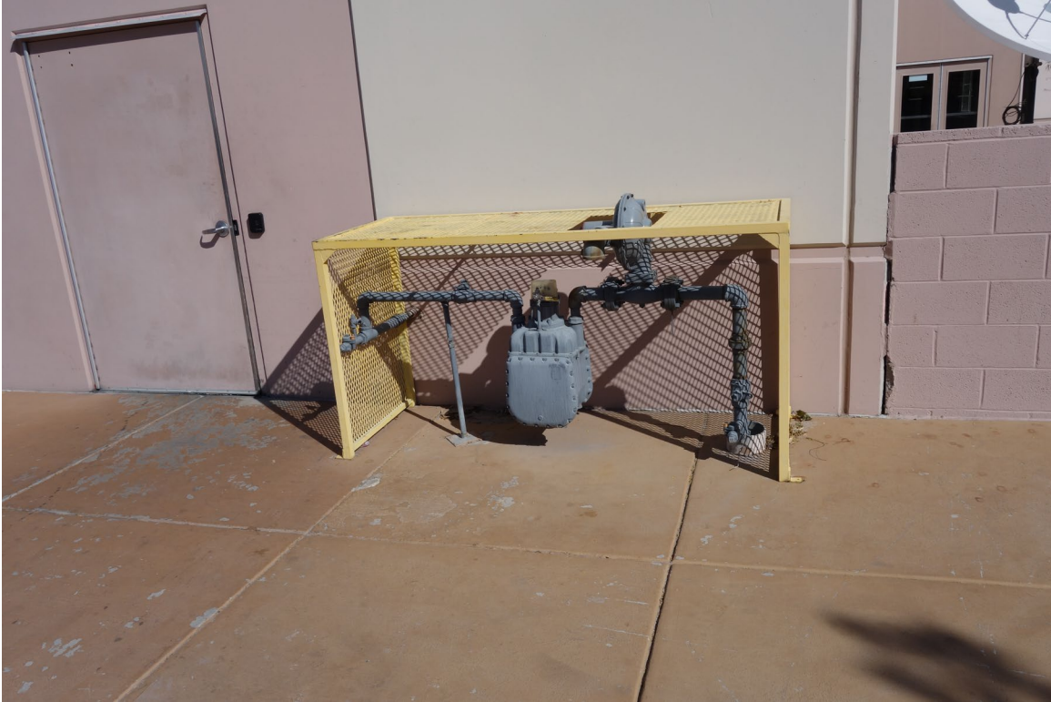
Administration Building – FCA Building #2559 Description: Seismic Gas Shut-Off Valve Needed.
