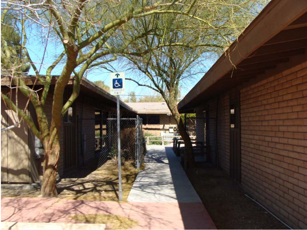
CNR Wildlife Offices Site - Site #9878 Description: ADA accessible route to the office.
