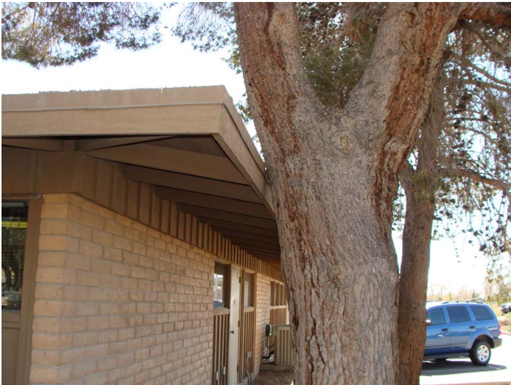
NDOW Regional Office - Building #0260 Description: Area of proposed roof modifications.
