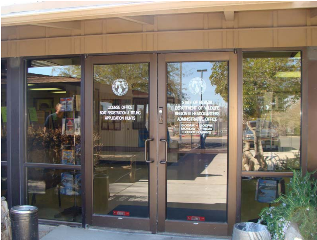
NDOW Regional Office - Building #0260 Description: Public entrance.
