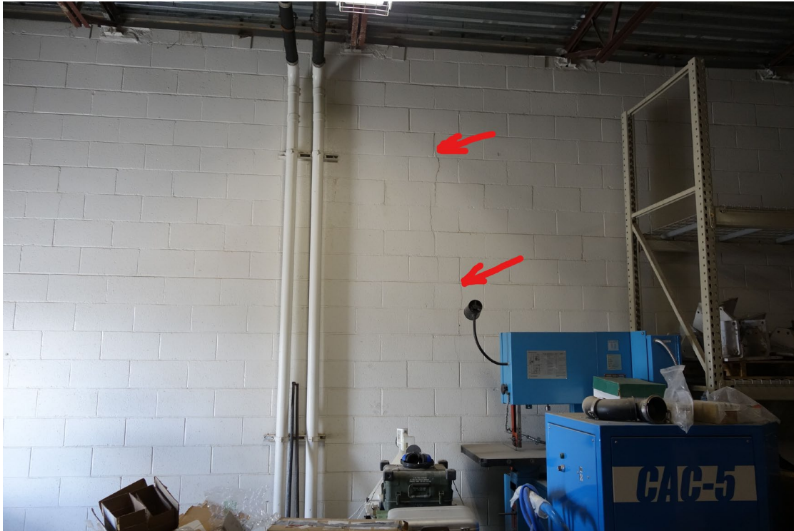
FETC CSMS Storage Building – FCA Building #1963 Description: Wall Crack #1 in CMU Wall.
