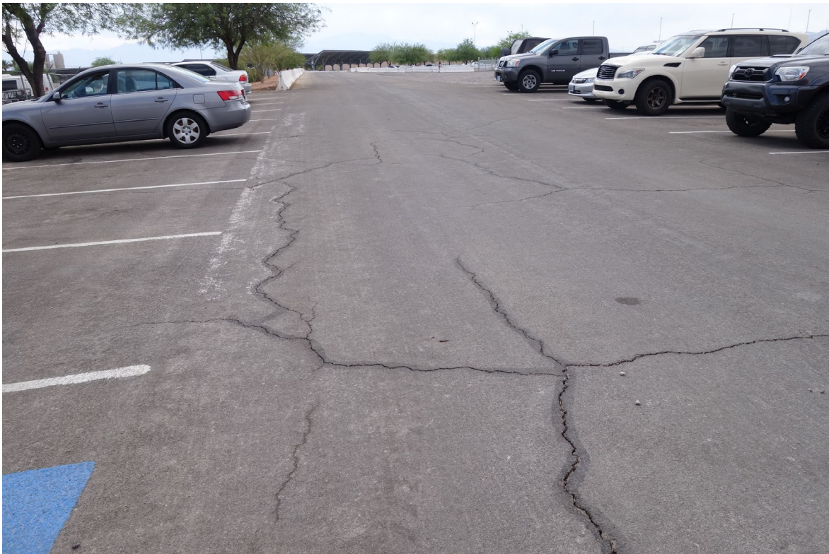
Floyd Edsall Training Center Site – FCA Site #9879 Description: Crack Fill & Seal Asphalt Paving.
