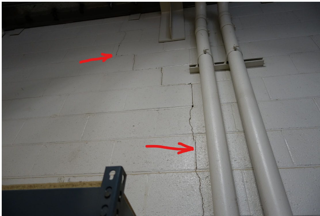
FETC CSMS Storage Building – FCA Building #1963 Description: Wall Crack #2 in CMU Wall.
