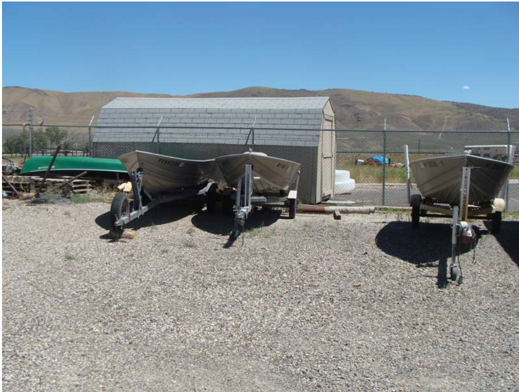
NDOW Storage Building - Building #2548 Description: Exterior of the structure.
