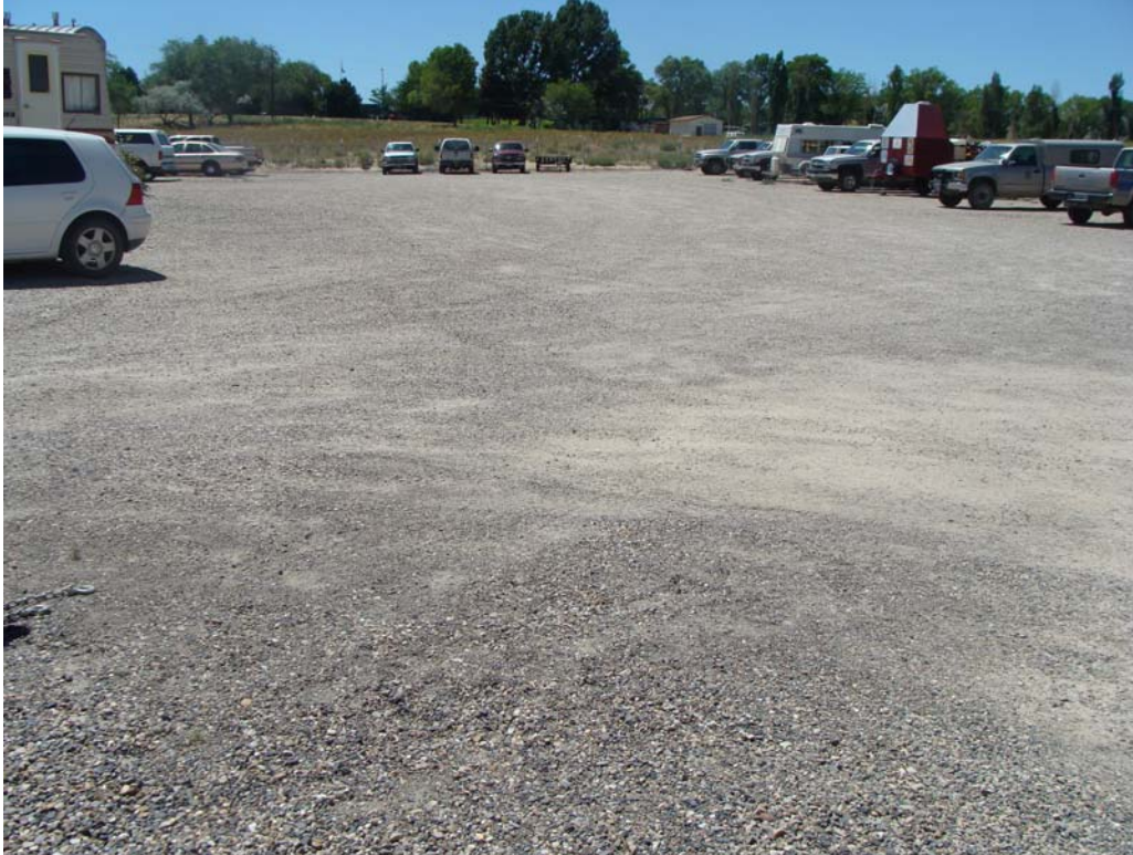
Eastern Regional Office Site - Site #9880 Description: Area of proposed A. C. paving installation.
