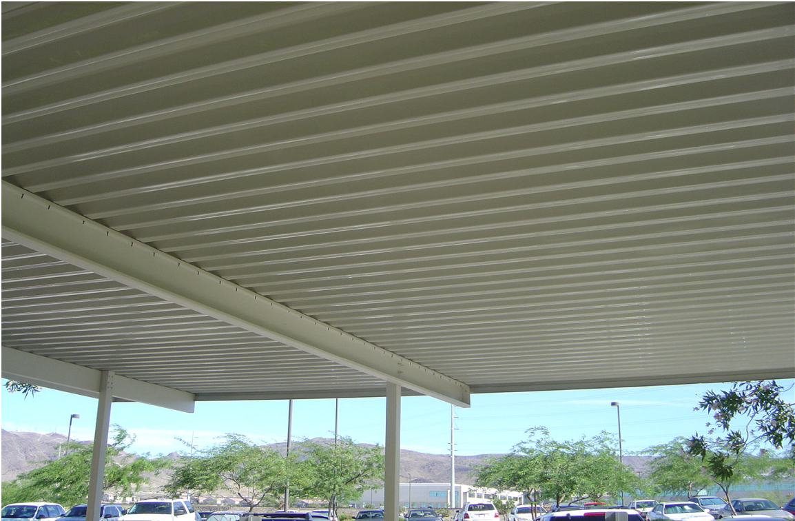
Shade Ramada - Building #2516 Description: View of the shade structure.
