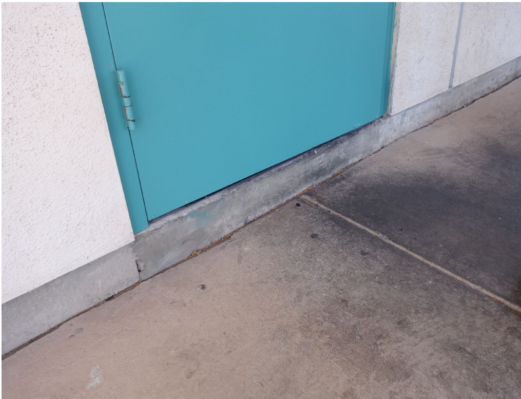
DMV Inspection Station - Building #2170 Description: Egress Door Landing Needed.
