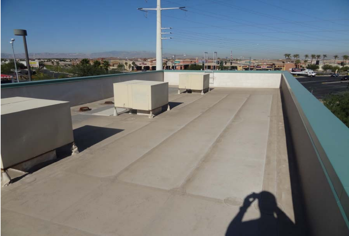
DMV Inspection Station - Building #2170 Description: View of the roof.
