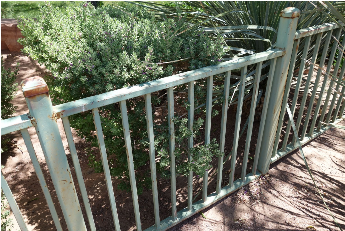
Henderson DMV Office Site - Site #9888 Description: Refinish Metal Fencing Needed.
