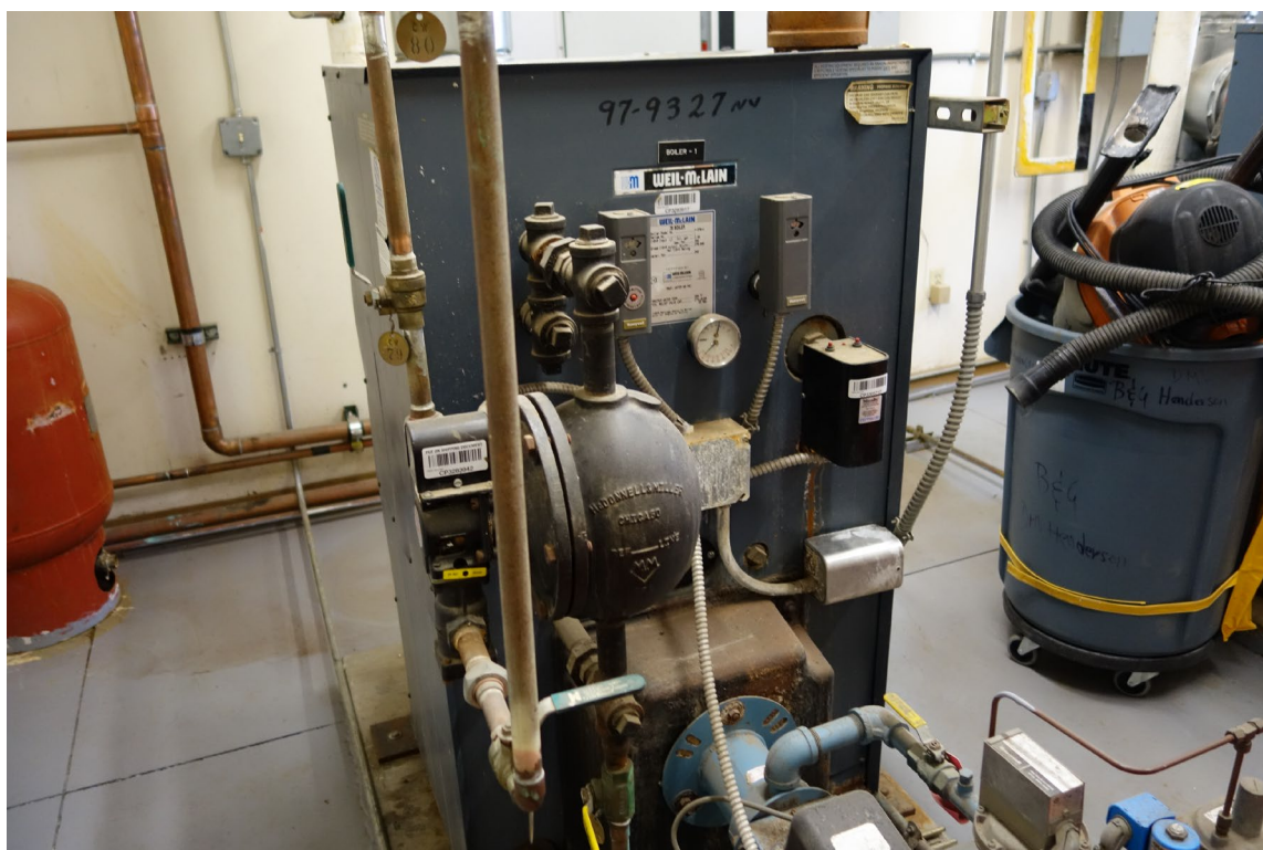
Henderson DMV Office - Building #2000 Description: Boilers Needing Replacement.
