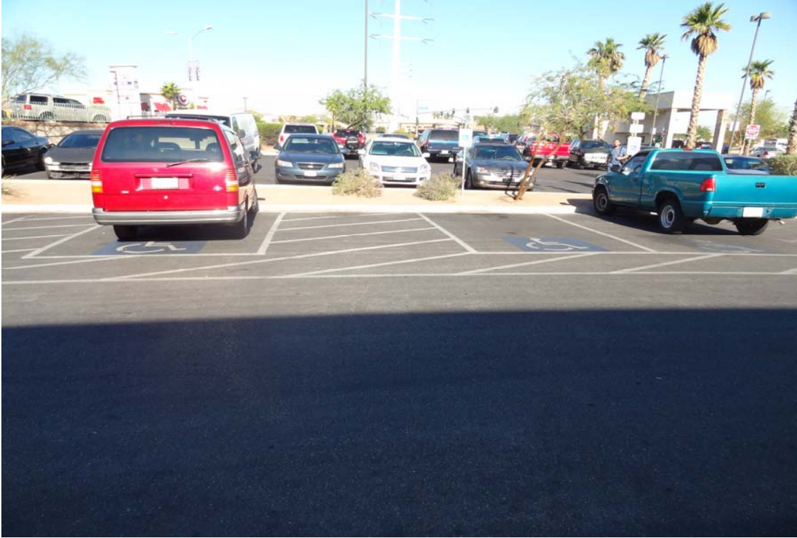
Henderson DMV Office Site - Site #9888 Description: View of ADA accessible parking.
