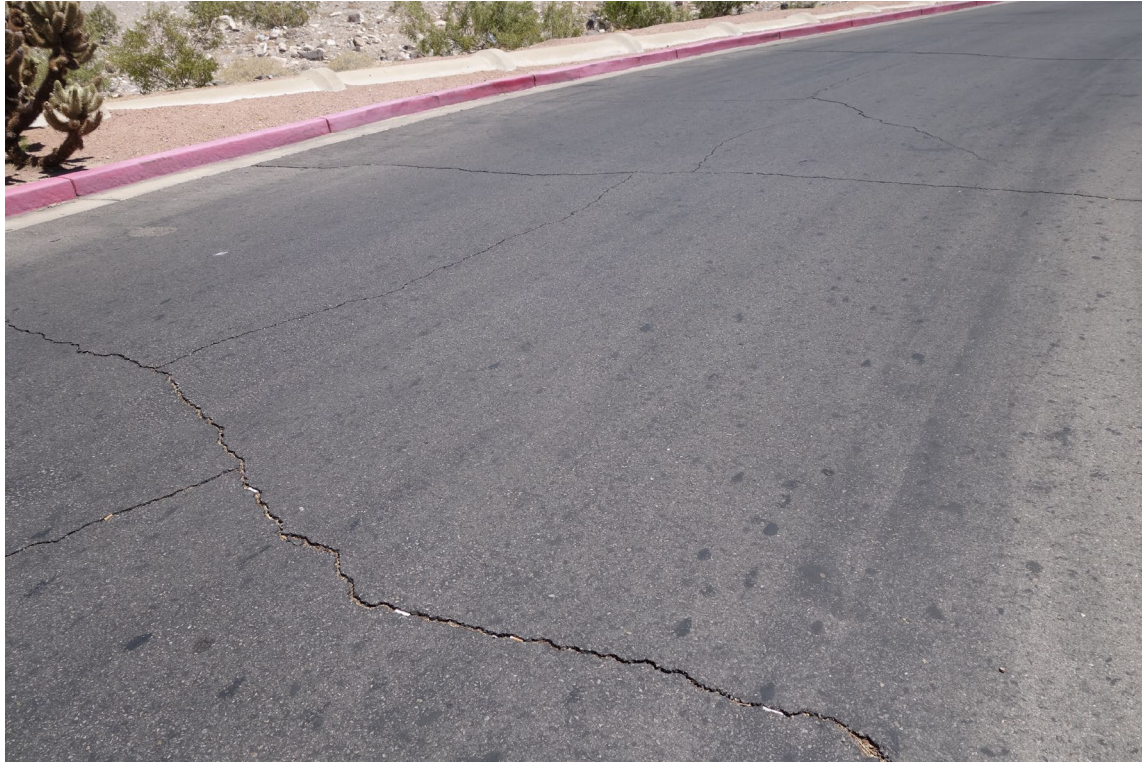
Henderson DMV Office Site - Site #9888 Description: Crack Fill & Seal Needed.
