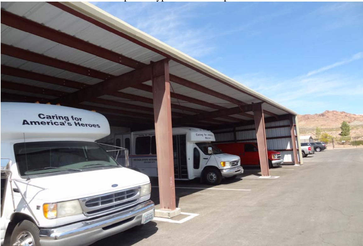
Vehicle Shade Structure - Building #3112 Description: Exterior of the structure.
