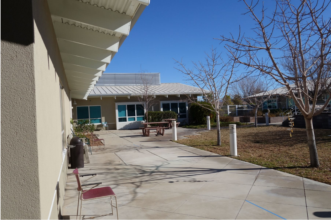
Southern Nevada Veterans Home – FCA Building #2106 Description: Typical Residence Patio Area.
