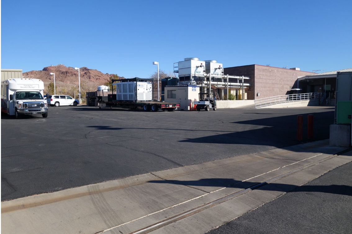
Southern Nevada Veterans Home Site – FCA Site #9889 Description: View of Loading Dock Area.
