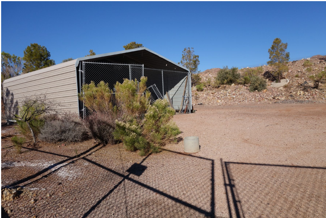
Storage Shelter – FCA Building #0614 Description: Exterior of the Structure.
