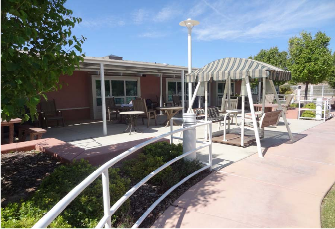
Southern Nevada Veterans Home Site - Site #9889 Description: Typical residence patio area.
