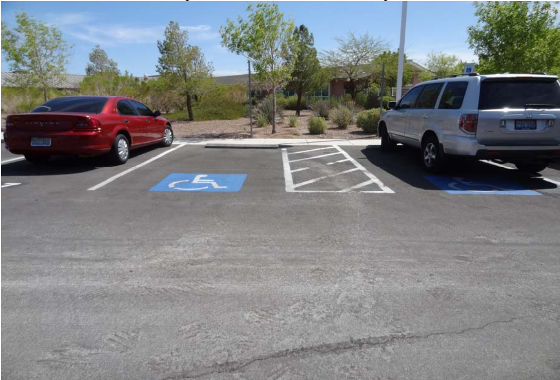
Southern Nevada Veterans Home - Building #2106 Description: ADA compliant Accessible parking.
