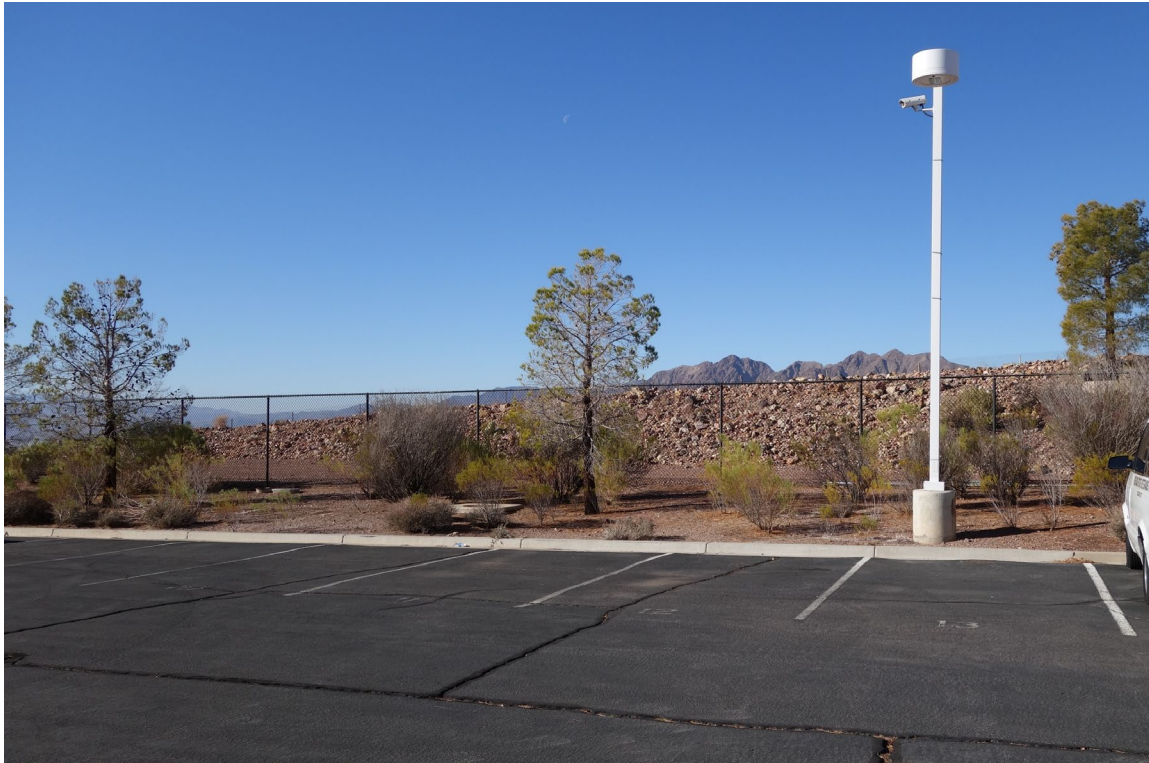
Southern Nevada Veterans Home Site – FCA Site #9889 Description: Video Surveillance Upgrade Needed.
