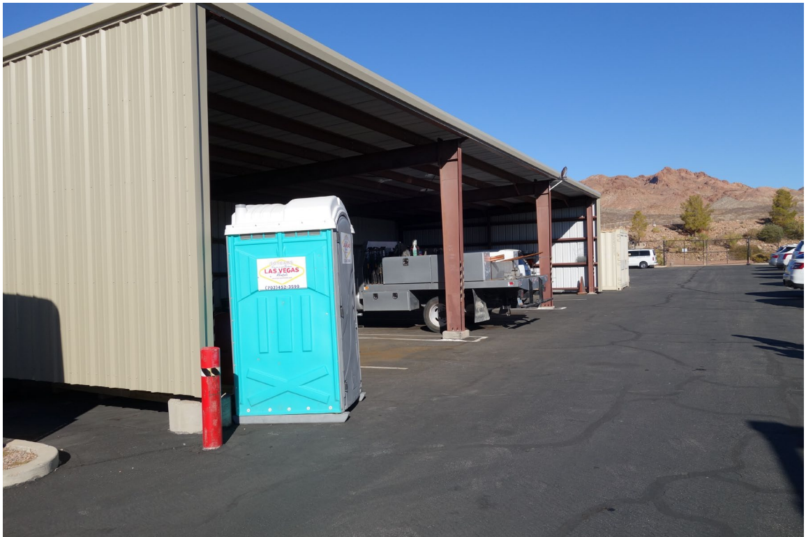
Vehicle Shade Structure – FCA Building #3112 Description: Exterior of the Structure.
