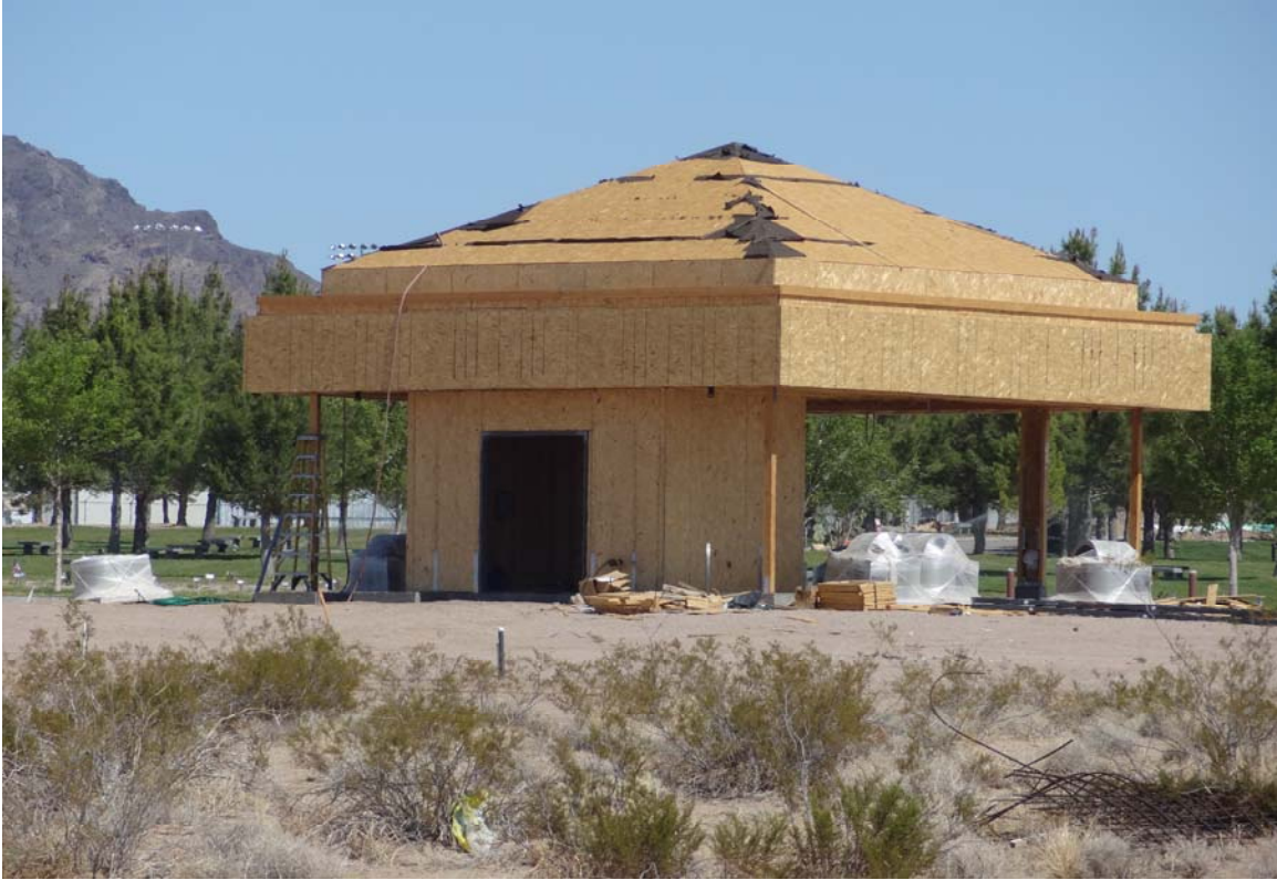
Outdoor Committal Building – FCA Building #3150 Description: Under construction.
