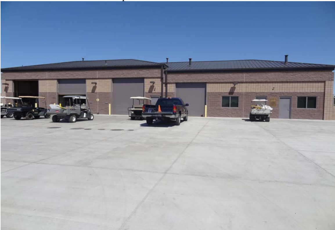
Maintenance / Office Building – FCA Building #2997 Description: Exterior of the building.
