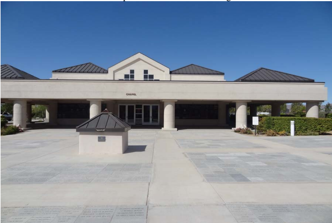
Chapel – FCA Building #2105 Description: Exterior of the building.
