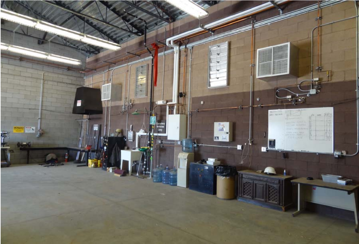
Maintenance / Office Building – FCA Building #2997 Description: Interior of the building.
