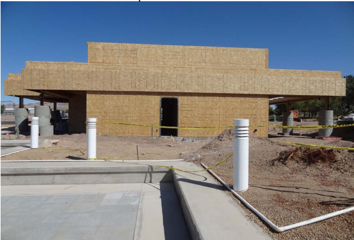
Administration Building – FCA Building #3147 Description: Under construction.
