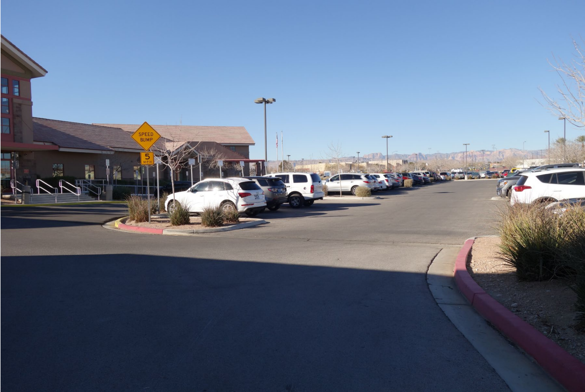
Rawson-Neal Psychiatric Hospital Site – FCA Site #9894 Description: View of the AC Paved Main Parking Area.
