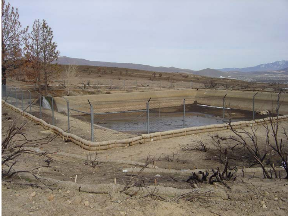
Marlette Lake / Ash Canyon - Building Index # 2486 Description: 1 Million Gallon Storage Reservoir
