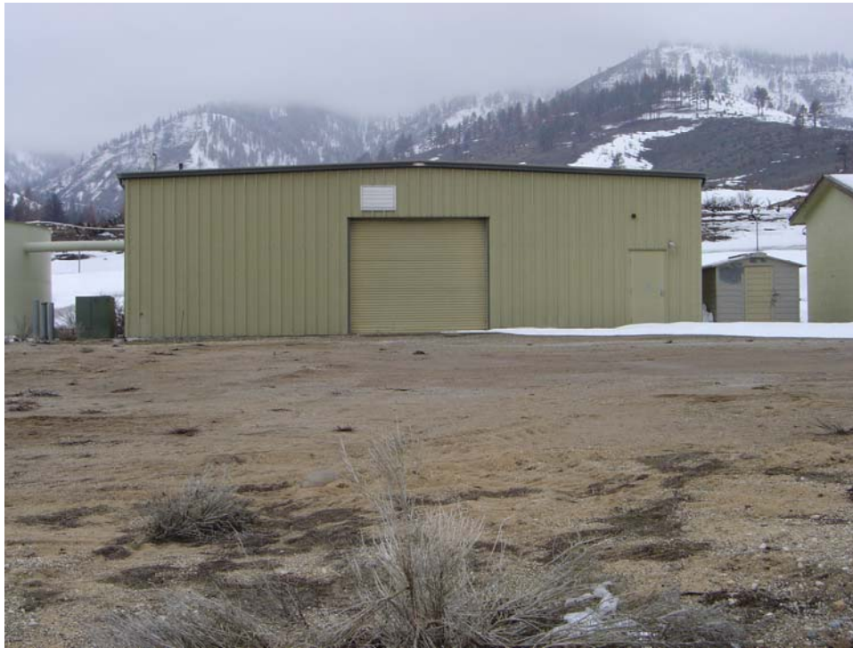
Marlette Lake / Ash Canyon- Building Index # 2487 Description: Marlette Lake Water Treatment Building
