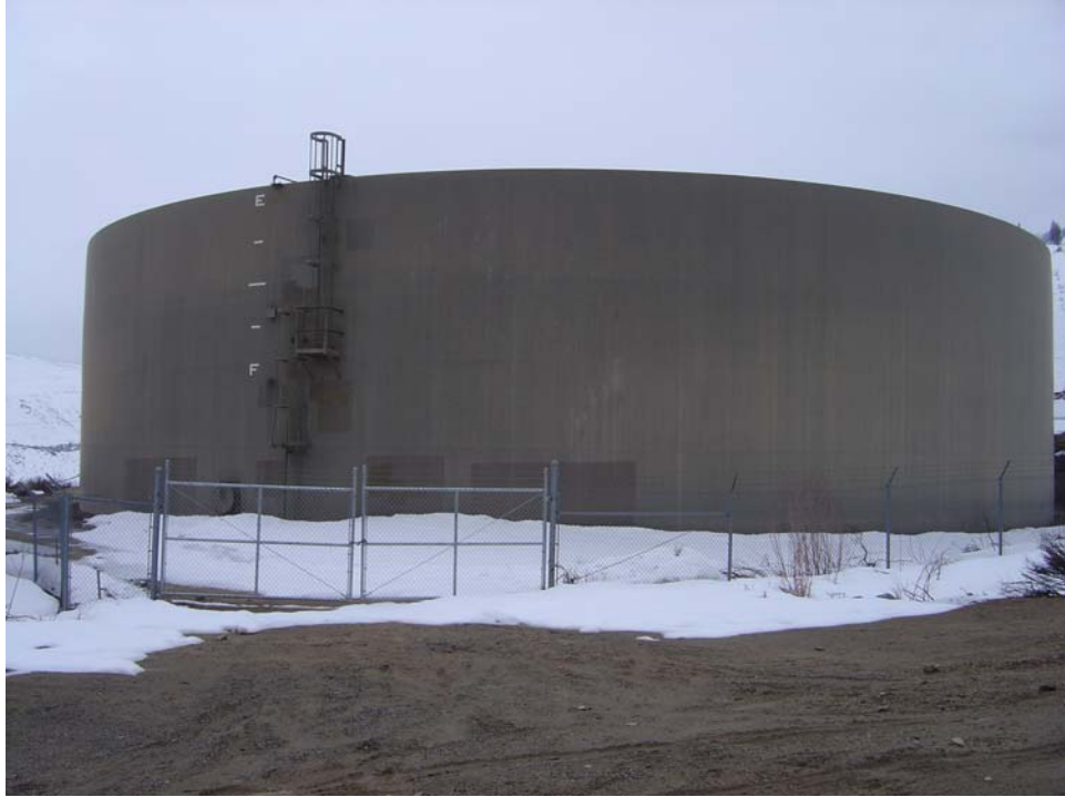
Marlette Lake / Ash Canyon- Building Index # 2485 Description: 3 Million Gallon Storage Tank
