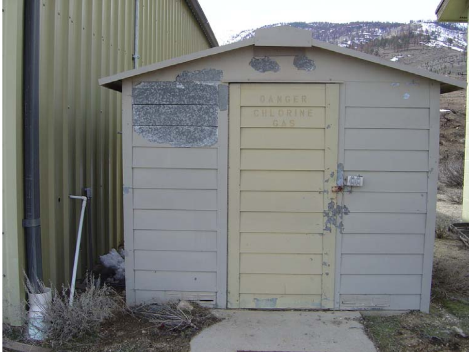
Marlette Lake / Ash Canyon- Building Index # 2503 Description: Marlette Storage Shed Exterior
