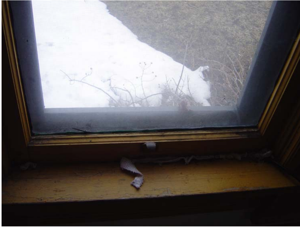
Marlette Lake Site – Building Number 2484 Description: Typical window sill.
