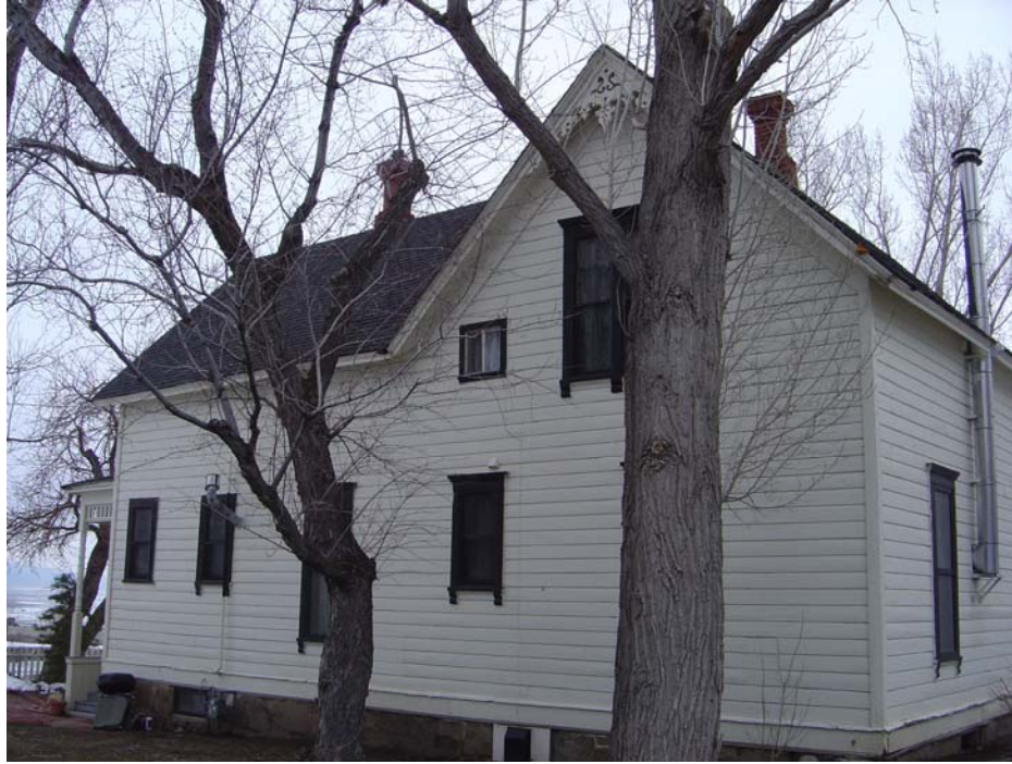
Marlette Lake Site - Building Number 2484 Description: Exterior of the Lakeview House.
