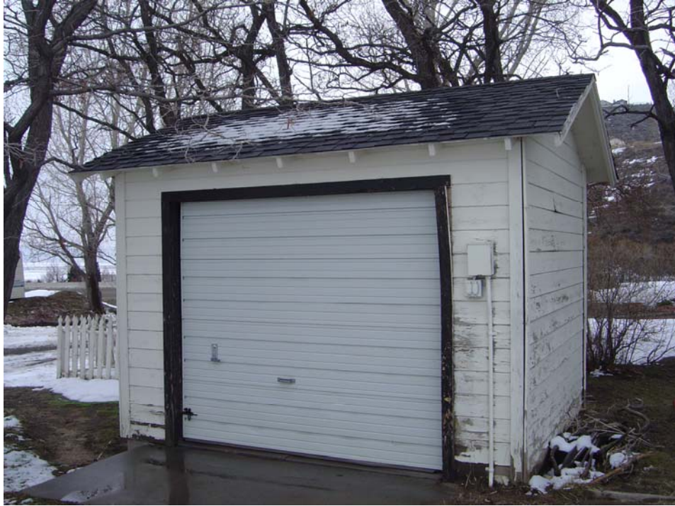
Marlette Lake Site - Building Number 2498 Description: Equipment shed.
