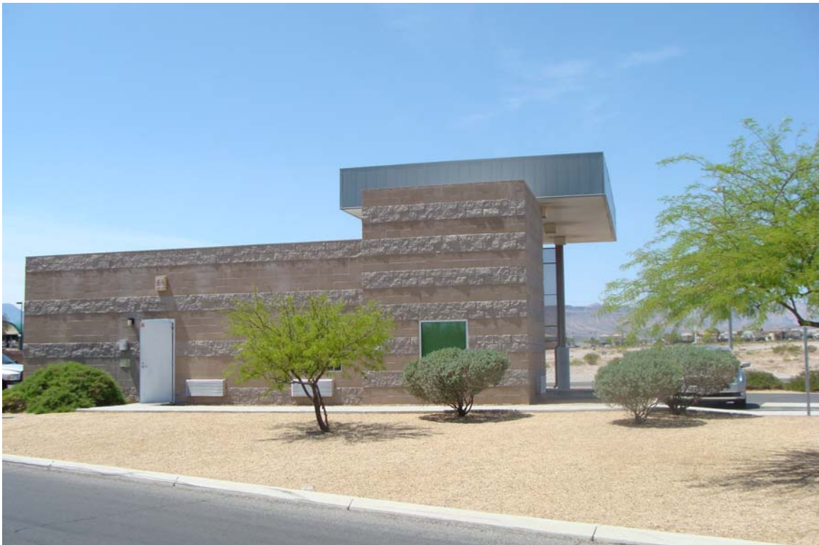
DMV Flamingo Inspection Station - Building #0366 Description: Exterior of the building.
