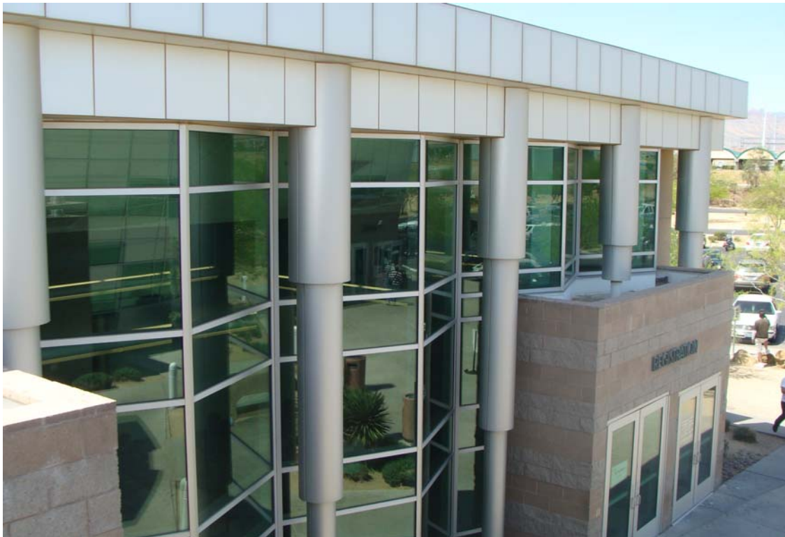
DMV Flamingo Office - Building #0338 Description: Glazed curtain walls.
