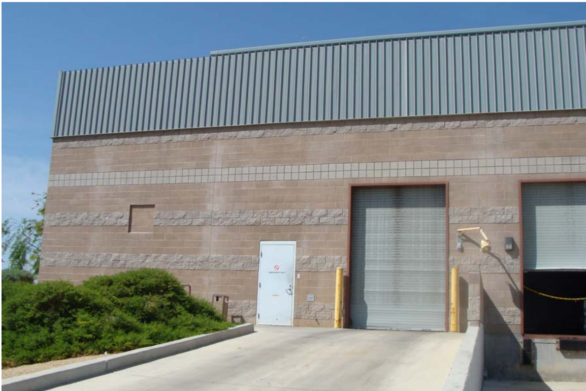
DMV Flamingo Warehouse - Building #0520 Description: View of loading dock area.
