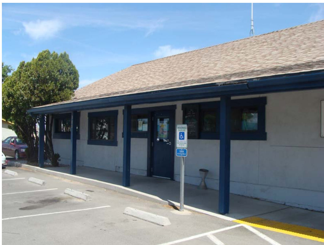
Field Office - Building #0633 Description: Exterior of the building.
