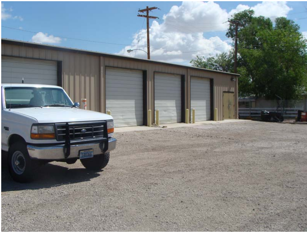
Boat Storage Facility - Building #1438 Description: Exterior of the building.
