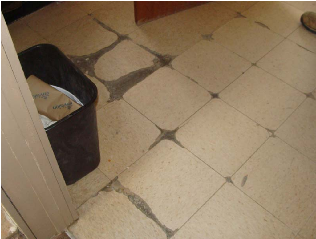
Mason Valley WMA Office / Headquarters - Building #0650 Description: Flooring in need of removal and replacement.
