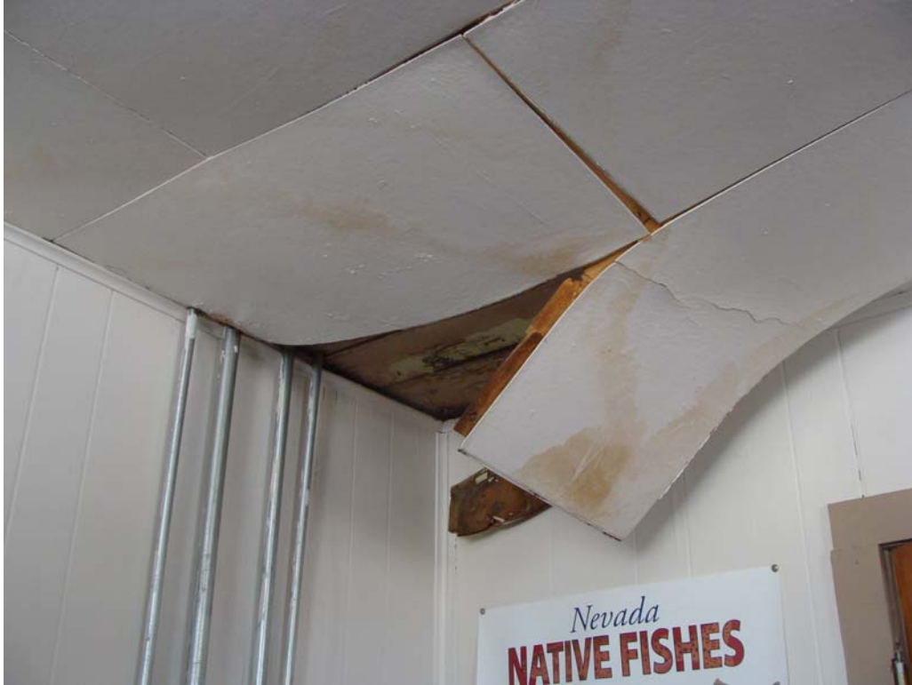
Mason Valley WMA Office / Headquarters - Building #0650 Description: Interior ceiling damage in office.
