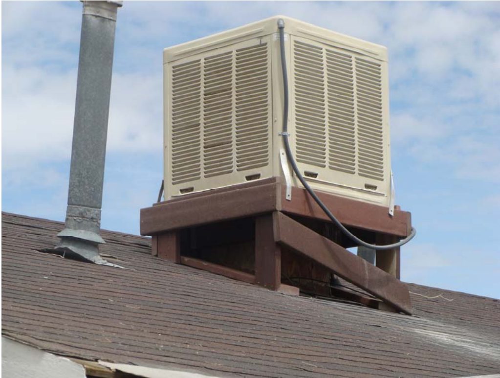
Mason Valley WMA Office / Headquarters - Building #0650 Description: Evaporative cooler and roof damage.
