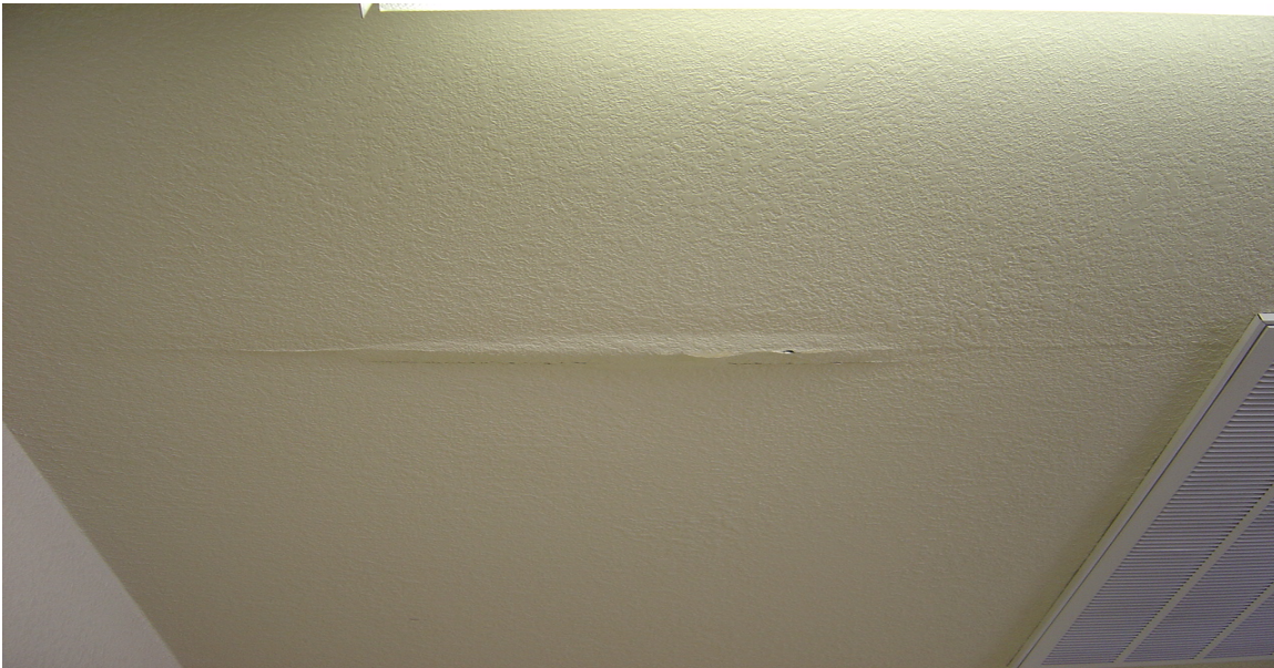
NDI in Las Vegas Site/NDI Office #2 - Building #2400 Description: Evidence of past roof leak.
