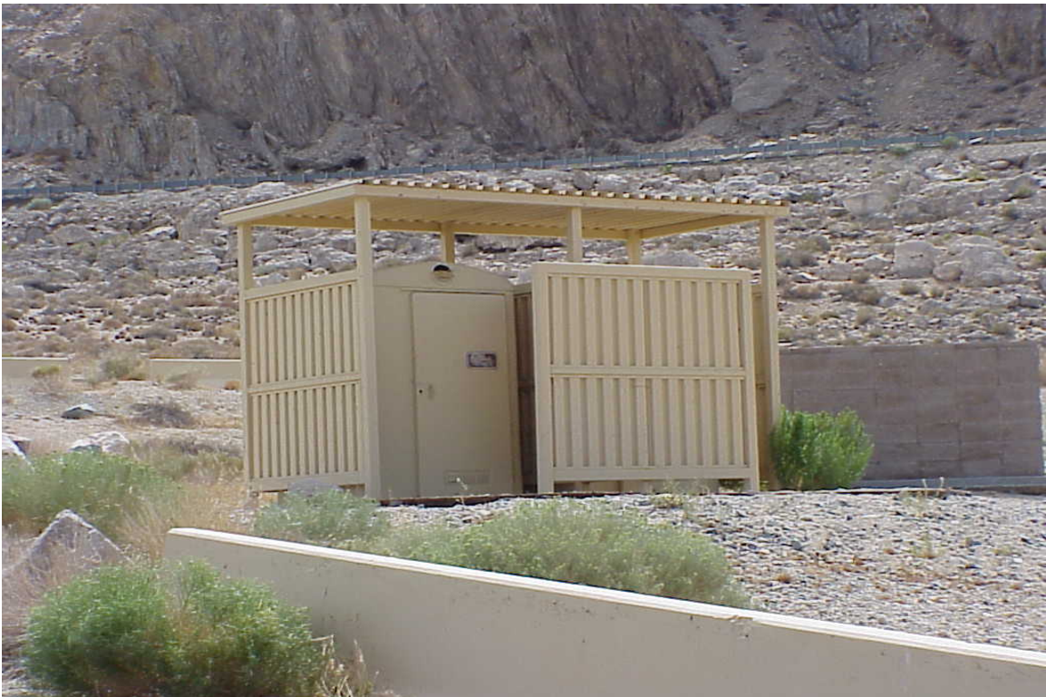
Walker Lake State Recreation Area Site #9915 Description: View of comfort station.
