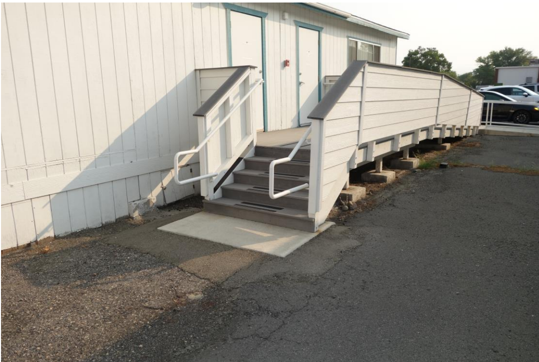
Education Modular Office-West - Building #2308 Description: Strengthen Guardrail.
