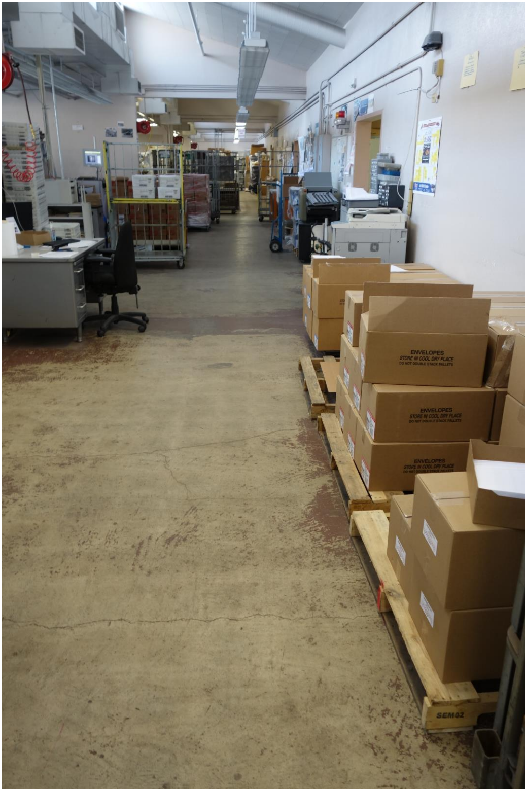
State Mail Services Building - Building #0395 Description: Resurface Concrete Floor.
