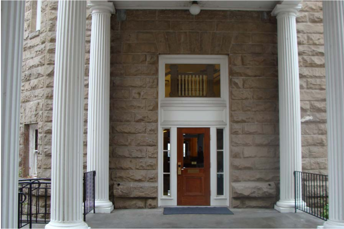
Nevada State Capitol Annex - Building #0203 Description: Public entrance.
