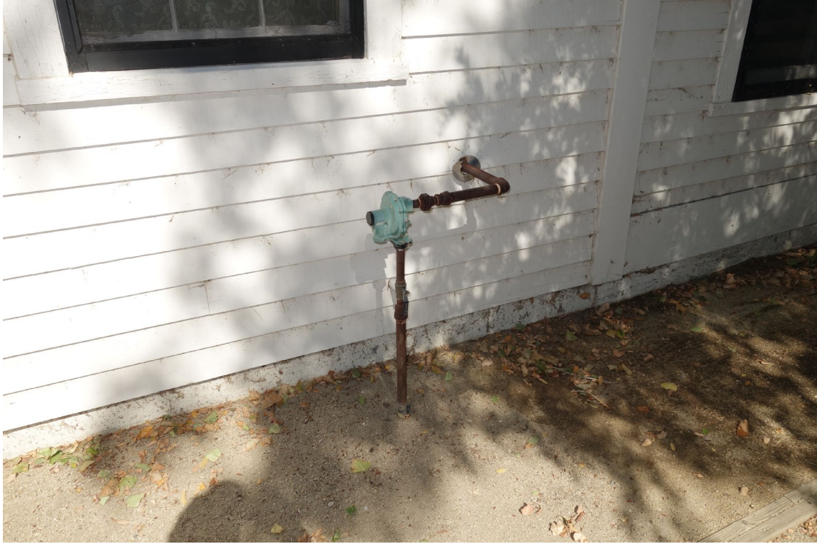
Buckland Station Historic Building - Building #0541 Description: Seismic Gas Valve Needed.
