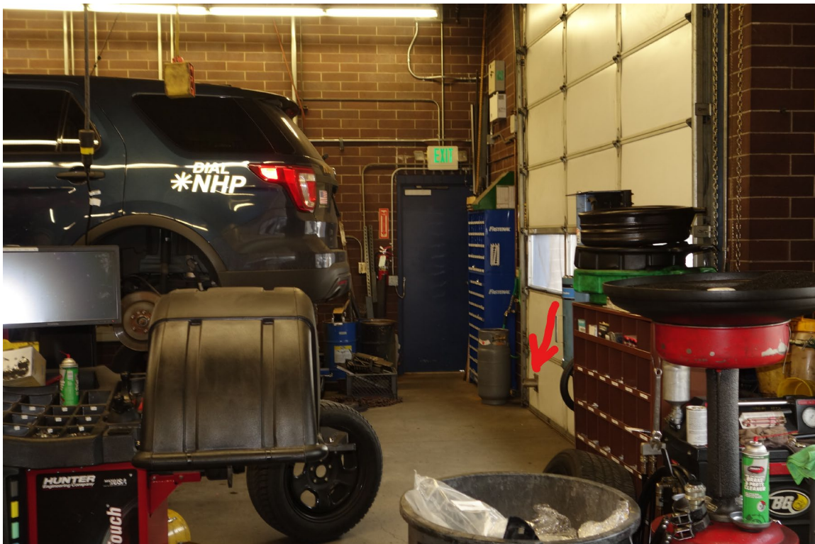
Regional Headquarters Garage / Shop - Building #1682 Description: Inadequate Vehicular Exhaust System (Red Arrow).
