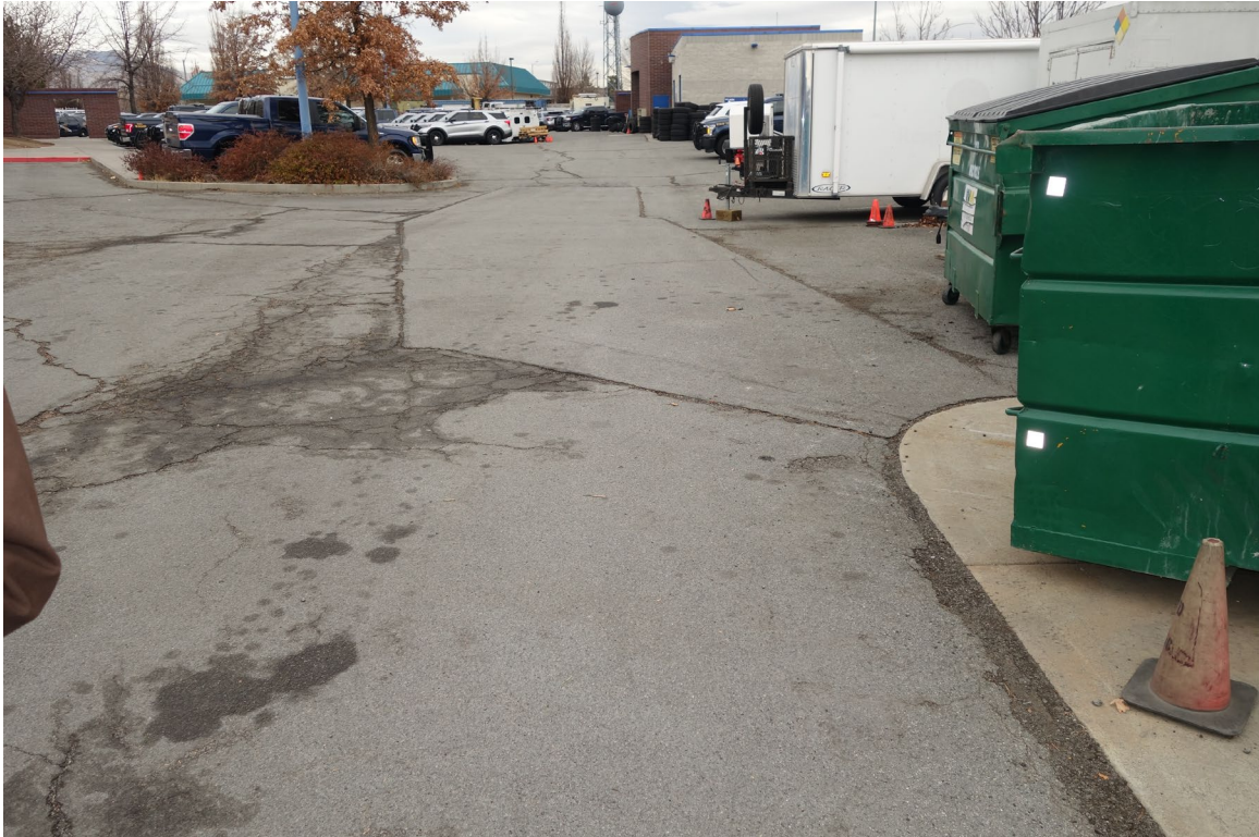
Reno NHP Headquarters Site - Site #9923 Description: AC Paving Patch, Crack & Slurry Seal Needed.
