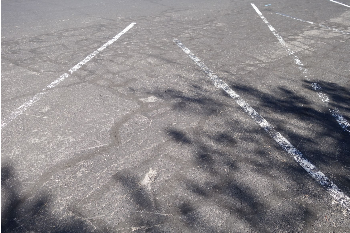
Lake Tahoe Nevada State Park – Cave Rock Site – FCA Site #9926 Description: Paving Crack Fill & Seal.
