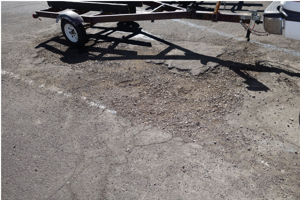
Lake Tahoe Nevada State Park – Cave Rock Site – FCA Site #9926 Description: Crack Fill & Seal - Paving Repair.
