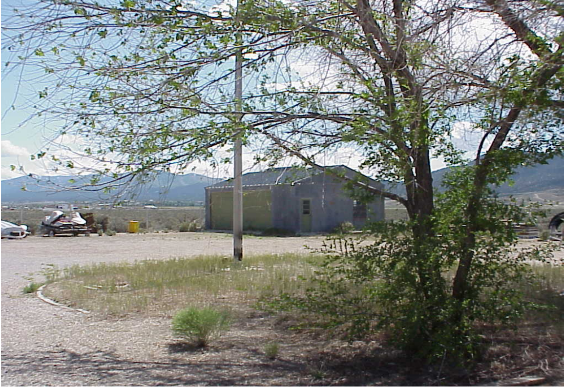
Division of Wildlife/Storage/Garage - Building #0636
