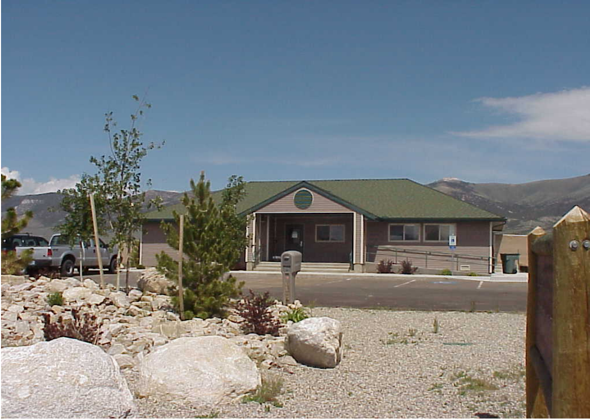
Wildlife Division/Ely Field Office - Building #2127 Description: The exterior of the building.
