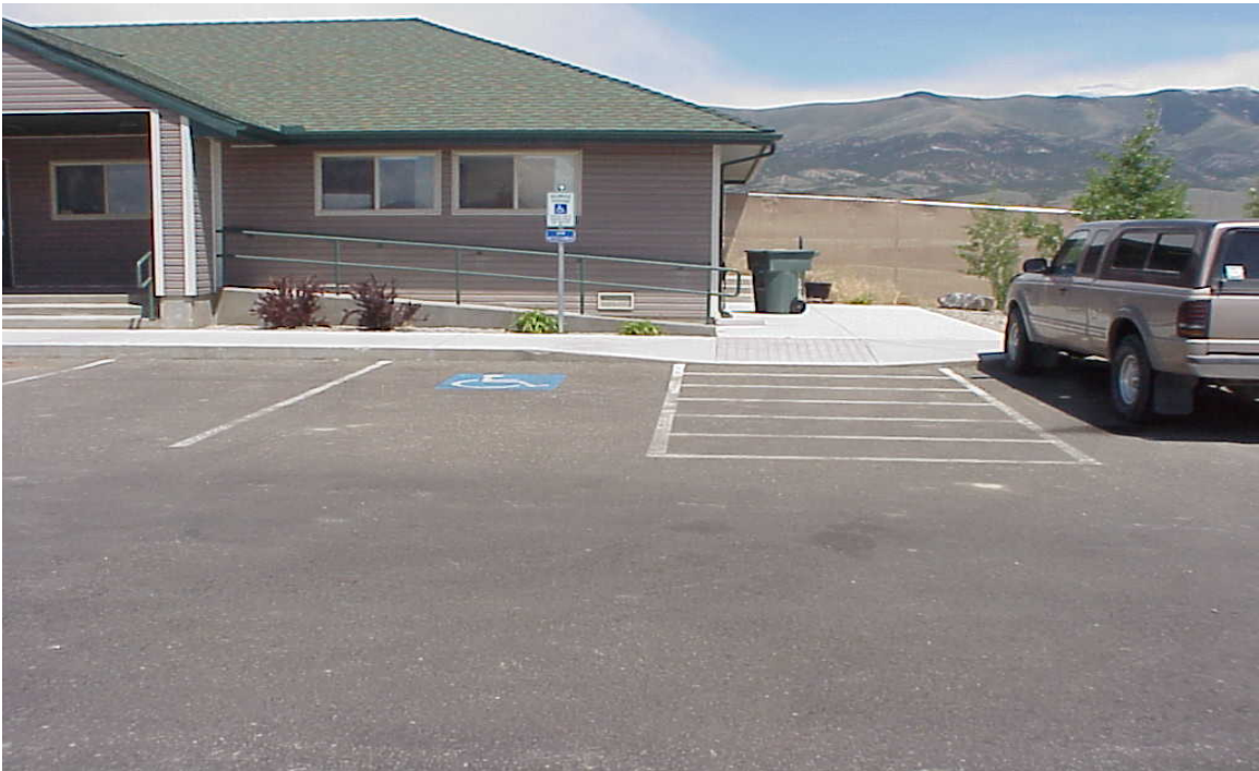
Wildlife Division/Ely Field Office - Building #2127 Description: ADA Parking.
