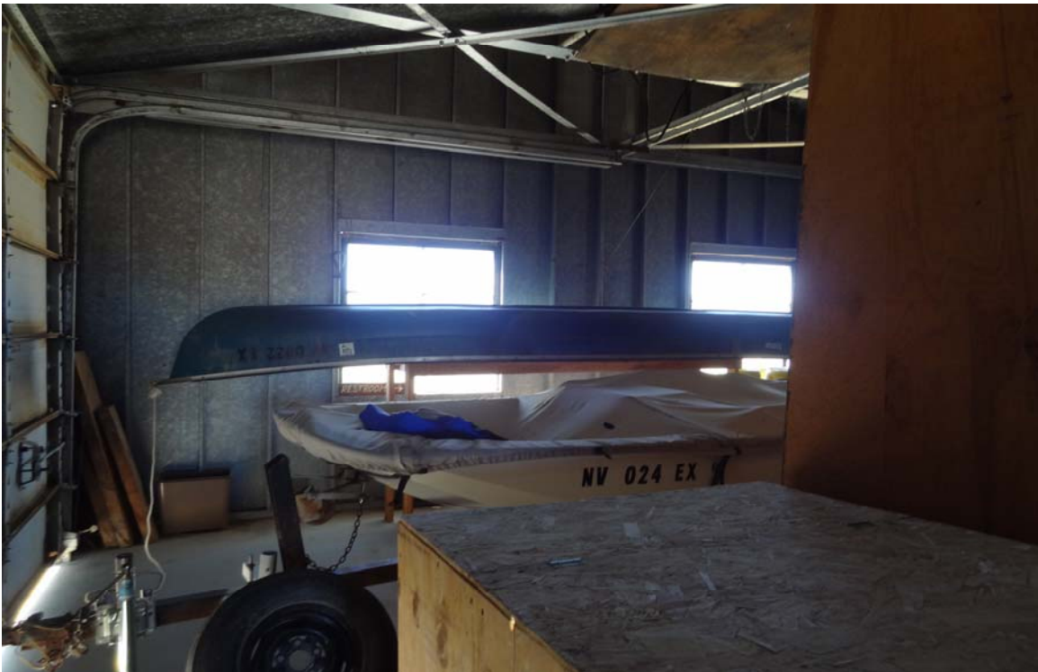
Wildlife Storage / Garage - Site #0636 Description: Interior of the building.
