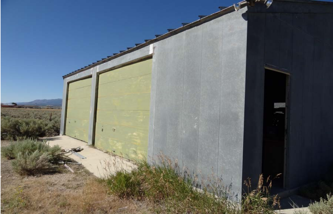
Wildlife Storage / Garage - Site #0636 Description: Exterior of the building.
