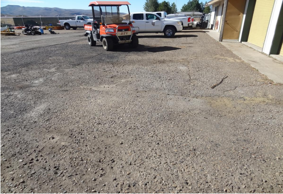
Wild Horse State Recreation Area Site – FCA Site #9935 Description: AC paving in need of removal and replacement.
